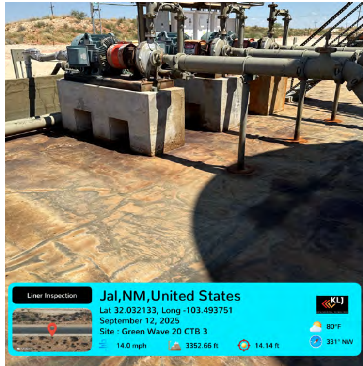
Liner under equipment on north side of containment.
