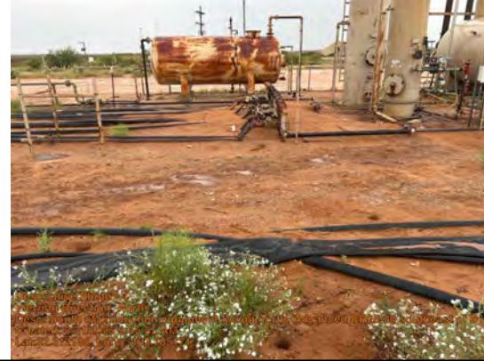
South of production equipment facing north. Advanced BH25-30 southeast of BH25-20.
