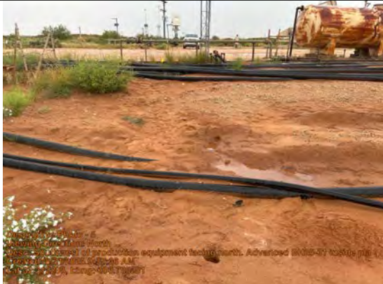
Southwest of production equipment facing north. Advanced BH25-31 inside planned remediation area for vertical delineation.
