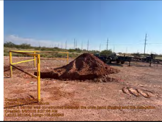
A barrier was constructed between the crew hand digging and the delegation hole to prevent falls
