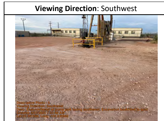
East-northeast of pump jack facing southwest. Excavation backfilled to grade.
