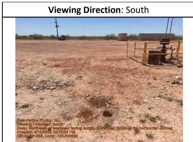
Northeast of wellhead facing south. Advanced BH23-15 for horizontal delineation.
