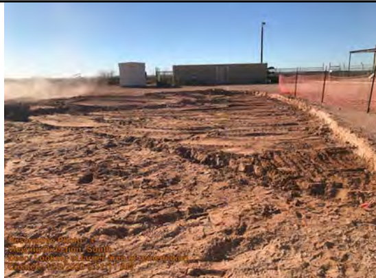
Looking at larger area of remediation.
