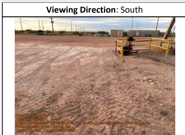
Northeast of pump jack facing south. Excavation backfilled to grade.
