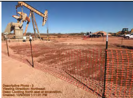
Looking North east at excavation.
