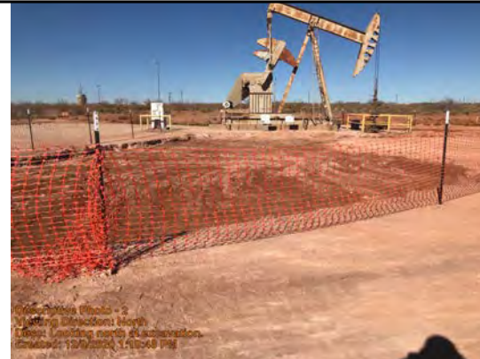
Looking north at excavation.
