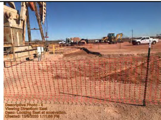
Looking East at excavation.
