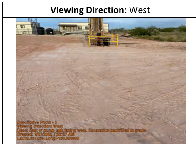
East of pump jack facing west. Excavation backfilled to grade.
