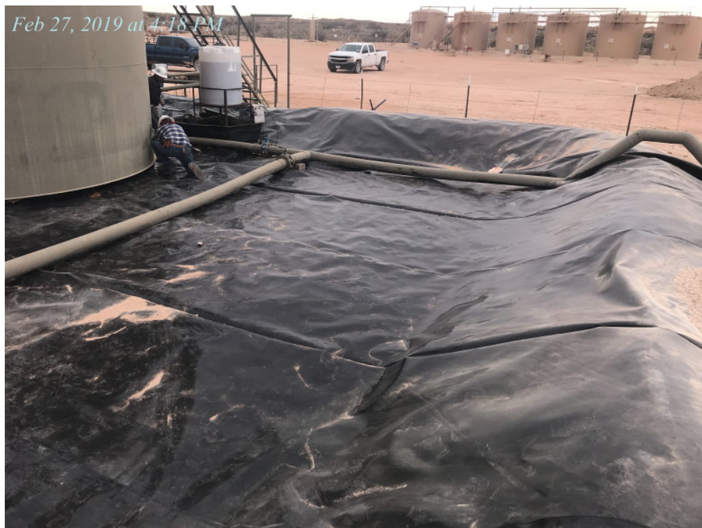
View South – Liner Installation
