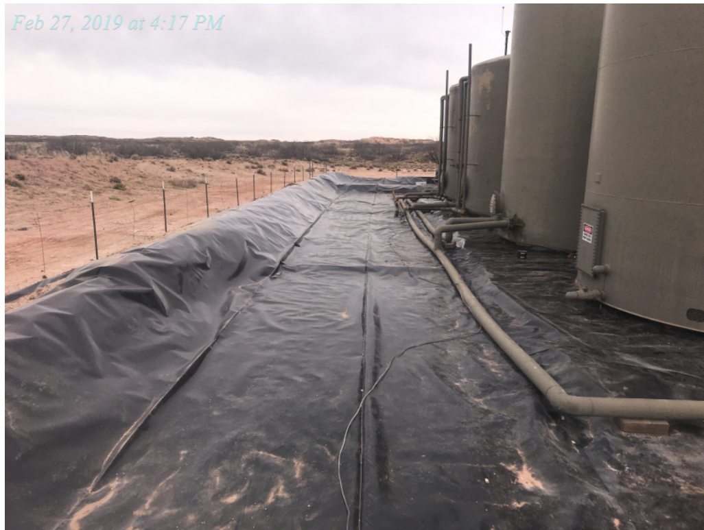
View East – Liner Installation
