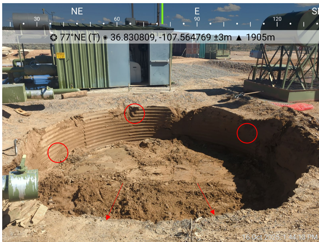
Photo 47: SS47 collected as a five-point composite confirmation sample from the sidewalls of the BGT following removal of the cellar.
