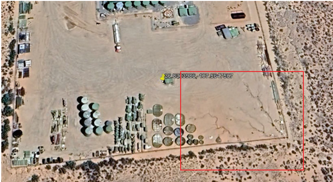
Photo 5: Erosion on southeast corner of facility.
