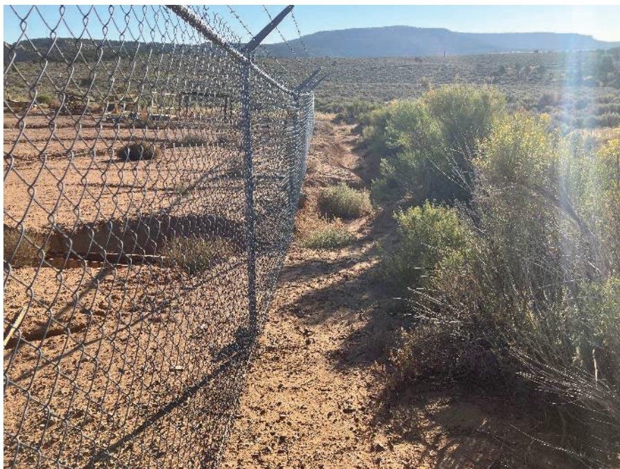
Photo 7: Erosion channel leaving facility in southeast corner.
