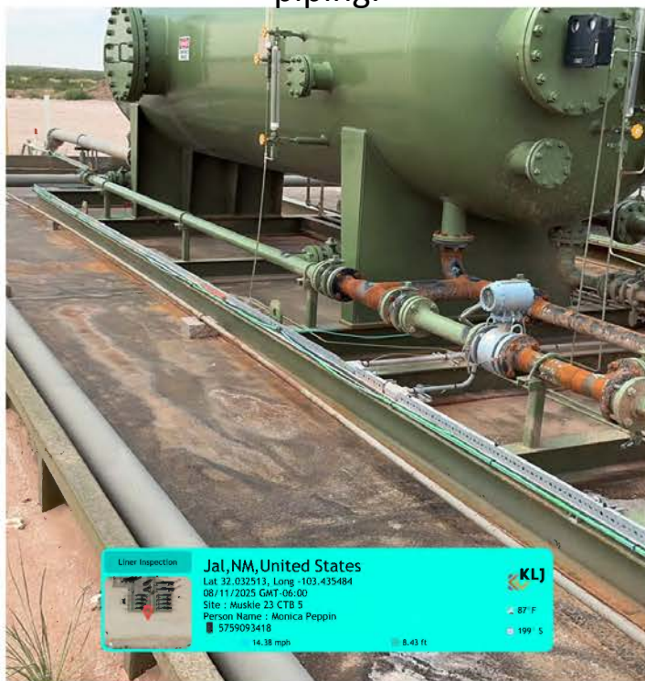
South view of liner on west side.
