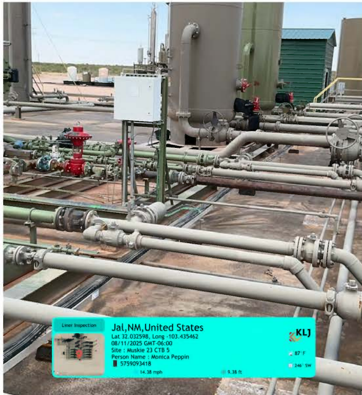
Facing northwest view of liner under piping.
