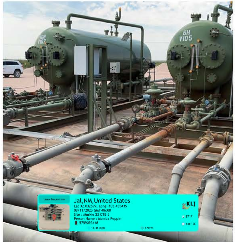
View of liner in southwest corner.
