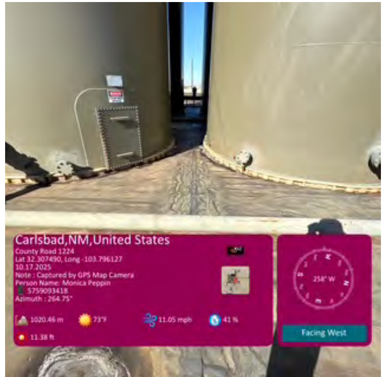
Liner between tanks from east side.
