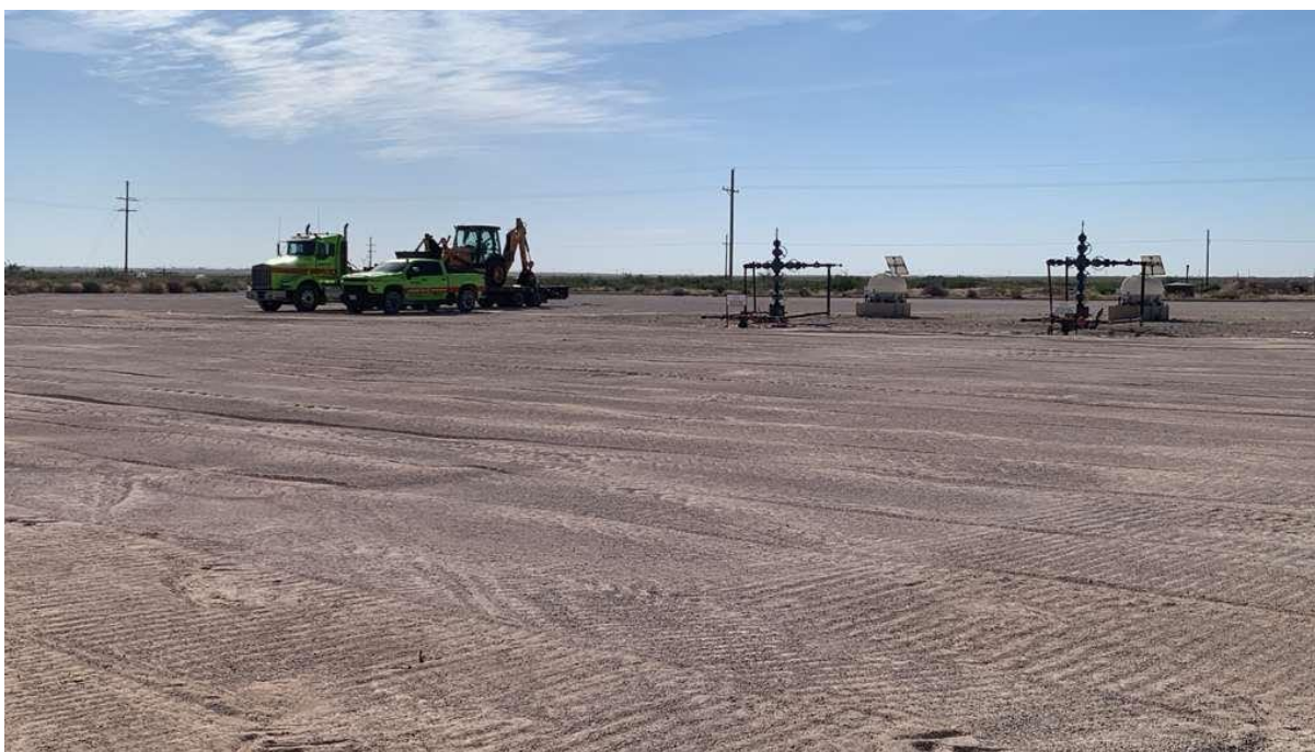
Caliche cap rolled, all waste off site
