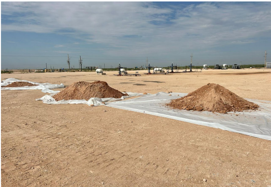
Stockpiling contaminated soil
