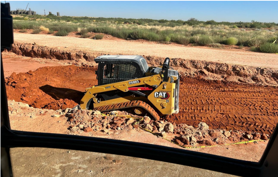
Further excavation of bottom hole after initial sample results
