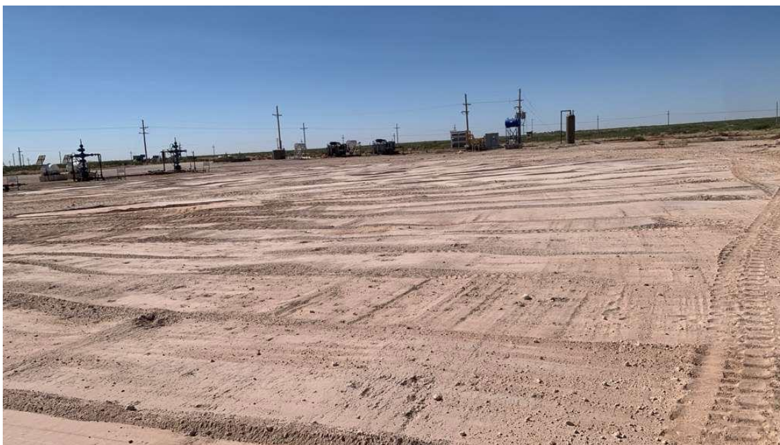
Back drag and leveling caliche cap
