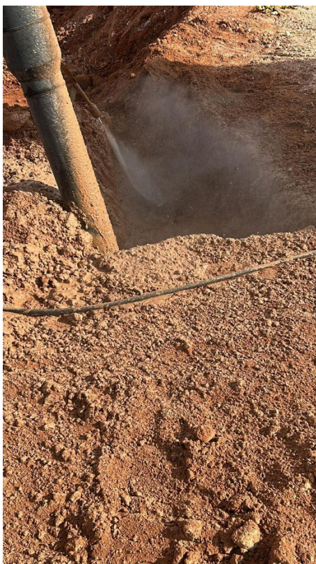
Hydro excavation near well heads
