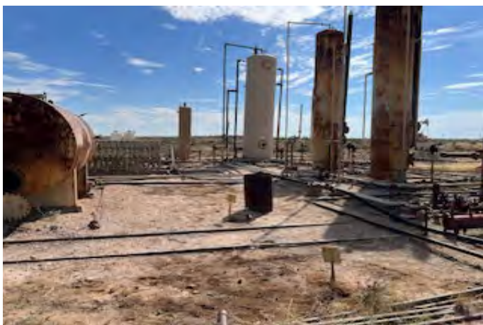
View to S of auger hole TH-19 (10/16/25).
