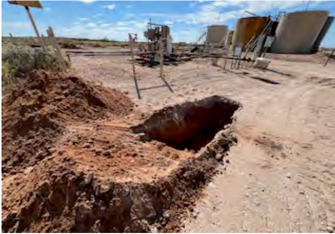
View to SW of test hole TH-23 (10/16/25).
