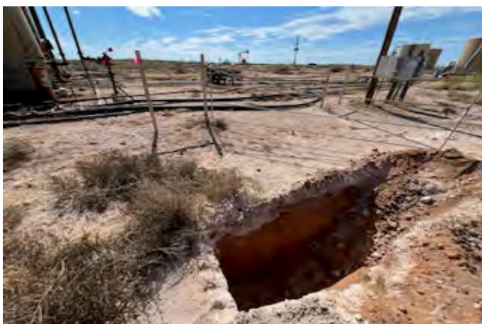
View to SW of test hole TH-21 (10/16/25).
