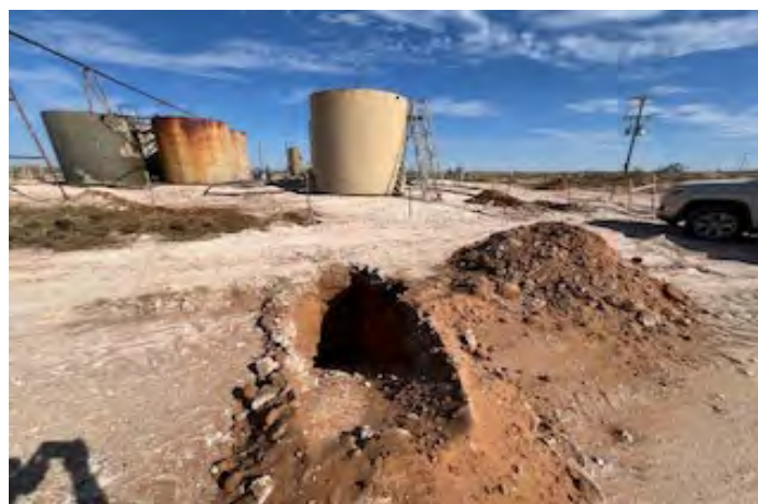
View to E of test hole TH-32 (10/16/25).
