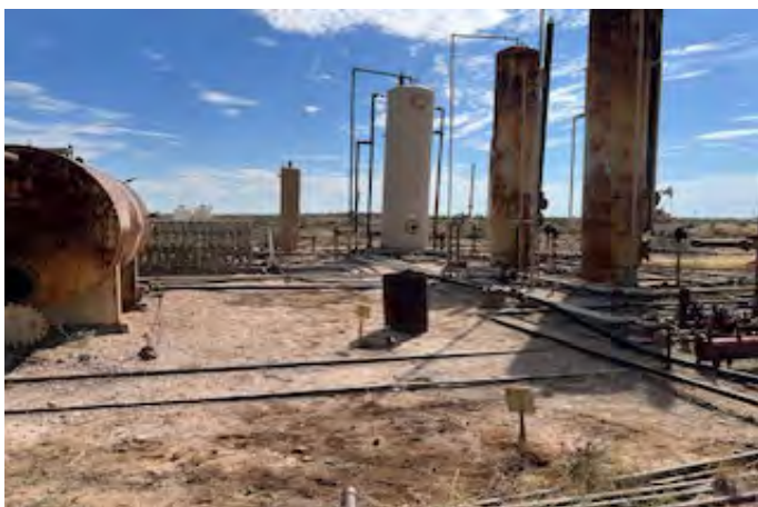
View to S of auger hole TH-19 (10/16/25).
