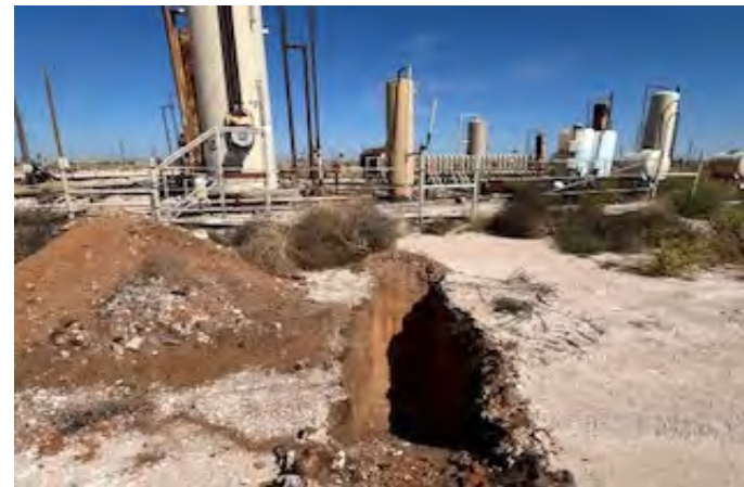
View to N of test hole TH-16 (10/16/25).
