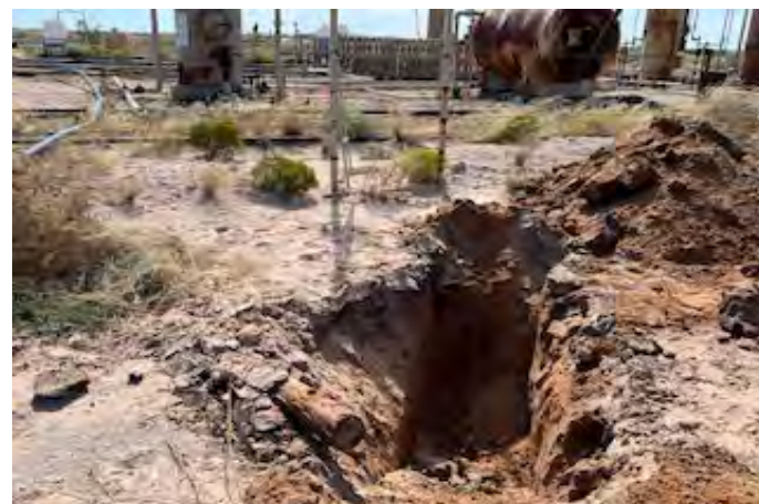
View to S of test hole TH-20 (10/16/25).
