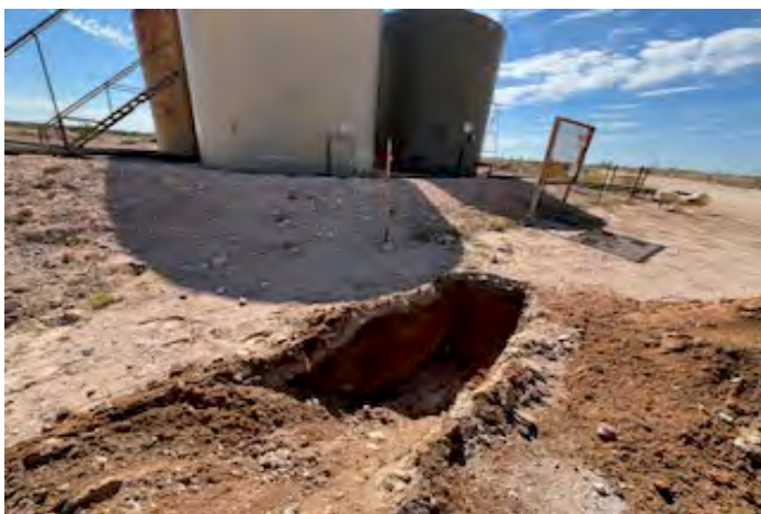
View to SW of test hole TH-31 (10/16/25).
