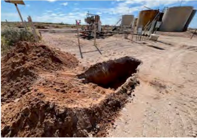
View to SW of test hole TH-23 (10/16/25).
