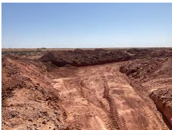
Photo #5 View toward south at over excavated remediation bench from north end. 4/10
