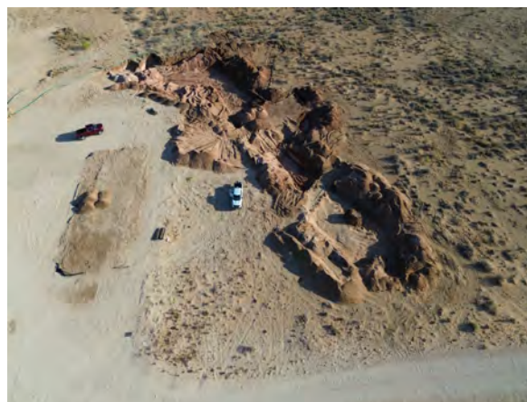
Photo #6 Aerial view looking north at over excavated remedial areas 4/10/25
