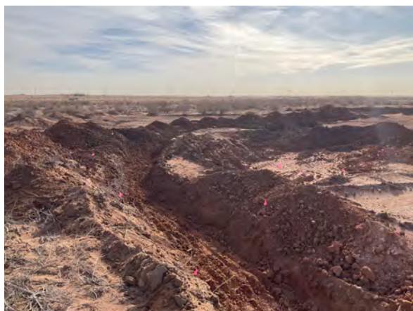
Photo #1 Initial trenching of impacted soils, east side on 3/3, view to SE
