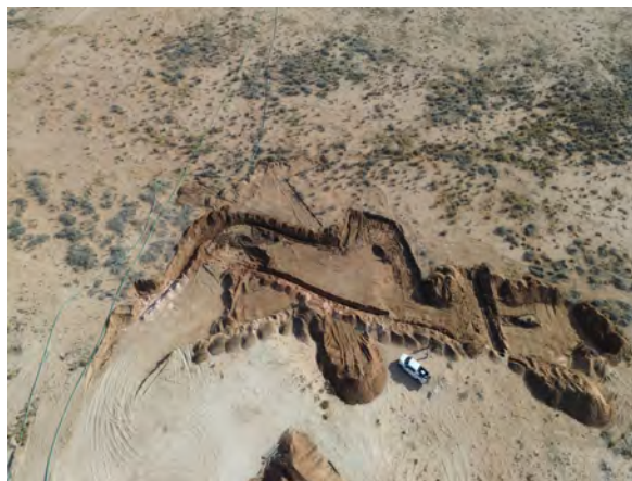
Photo #2 Aerial view to east of remediated area on 3/3.
