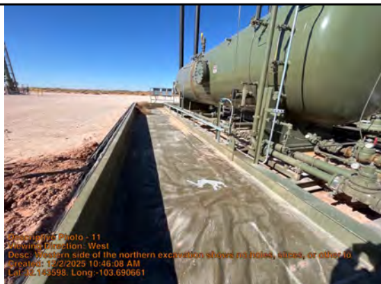
Viewing Direction: West
