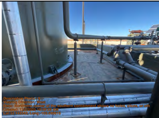
Viewing Direction: West
