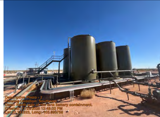
North side of the tank battery containment.
