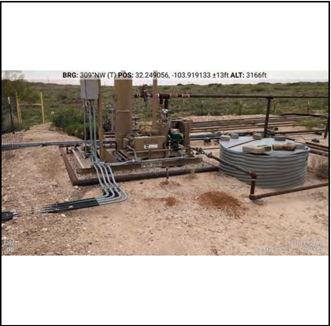
Photograph 4 Date: 05/14/2025 Description: BH21 View: Northwest
