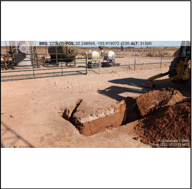
Photograph 2 Date: 02/05/2025 Description: SS07 View: North-northeast
