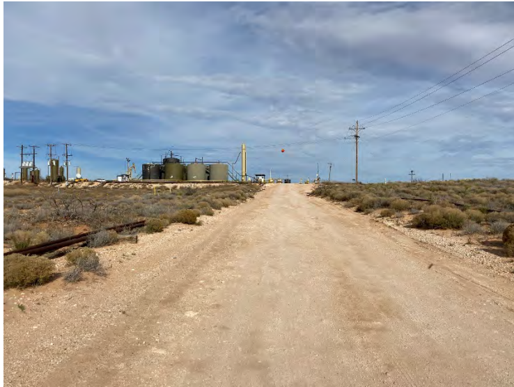
Photograph 1: View of lease road leading to pad – looking east.
