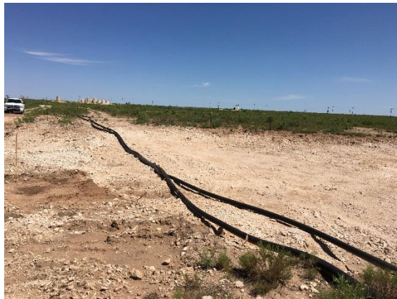
Excavated area with 3' of lines
