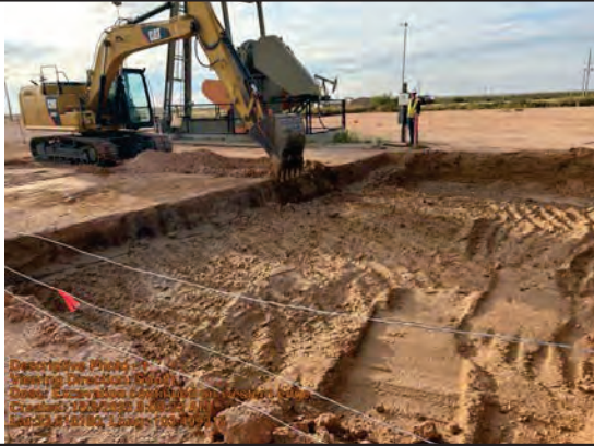
Excavation continued on western edge
