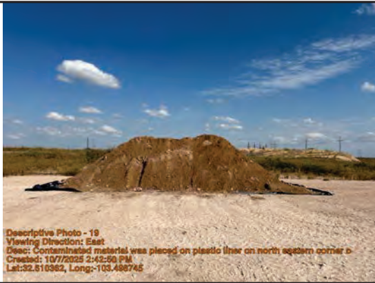
Contaminated material was placed on plastic liner on north eastern corner of pad
