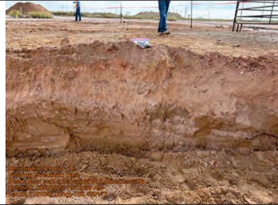
East wall excavation of 3' excavation
