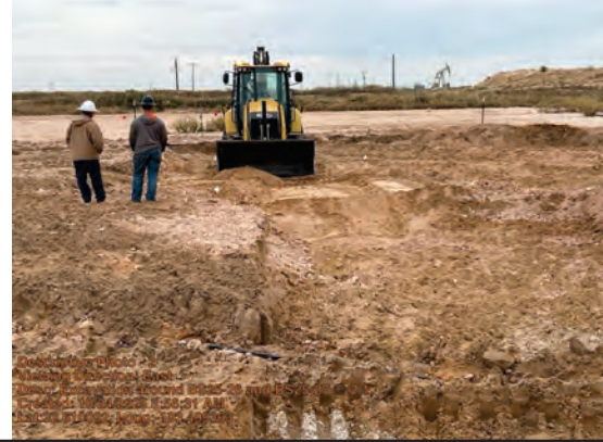
Excavation around BS25-26 and BS25-27 @ 2.1'
