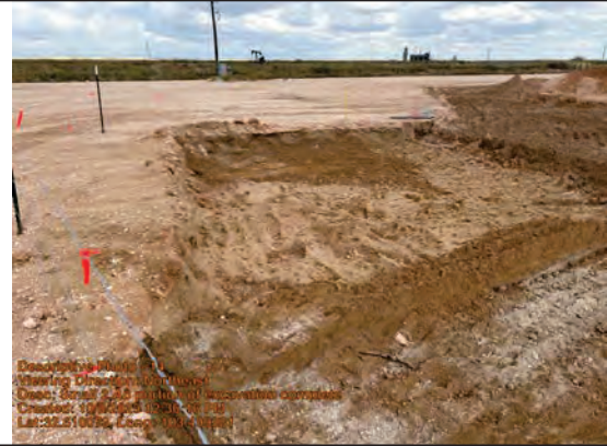
Small 2' portion of excavation completed
