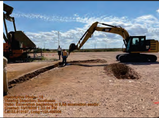
Excavation beginning in 3' excavation section
