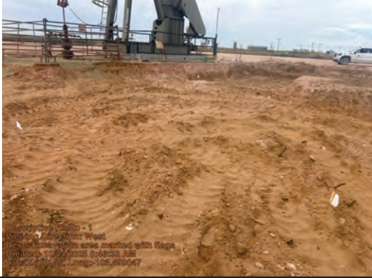
Excavation area marked with flags
