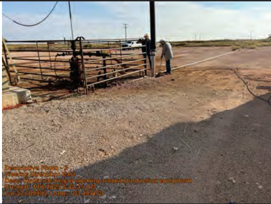
Hydrovac began working around production equipment
