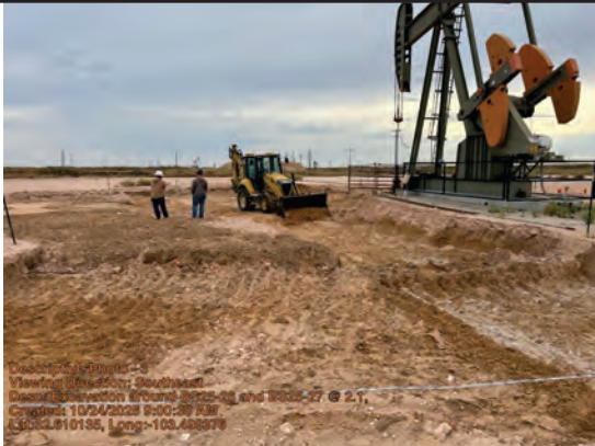
Excavation around BS25-26 and BS25-27 @ 2.1'
