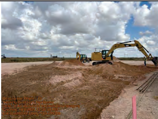
1' portion of excavation in progress
