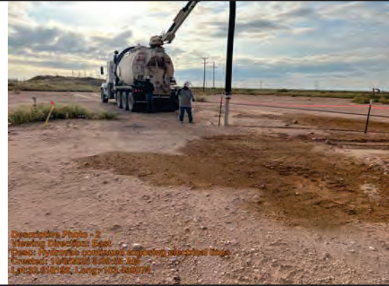
Hydrovac continued exposing electrical lines
