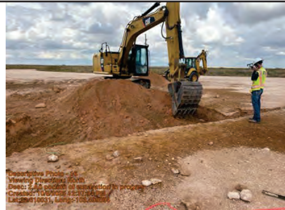
2' portion of excavation in progress
