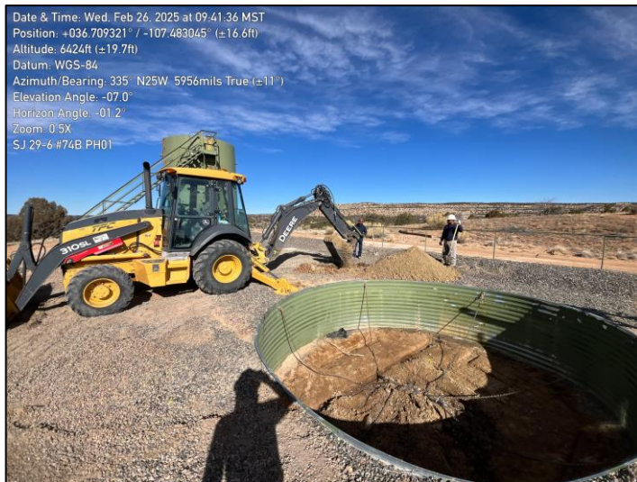
Photograph: 2 Date: 02/26/2025 Description: Backhoe Pothole Delineation Activities, PH01 View: North
