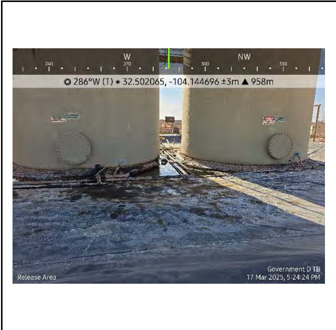
Photograph 4 Date: 3/17/2025 Description: Release Area View: West
