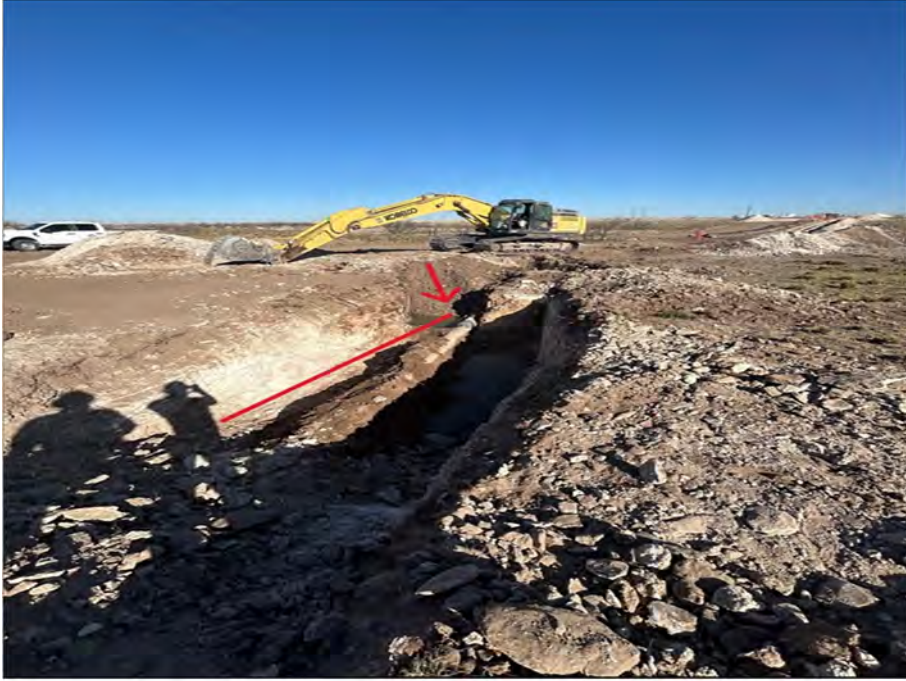
Pipeline Excavation Area:
