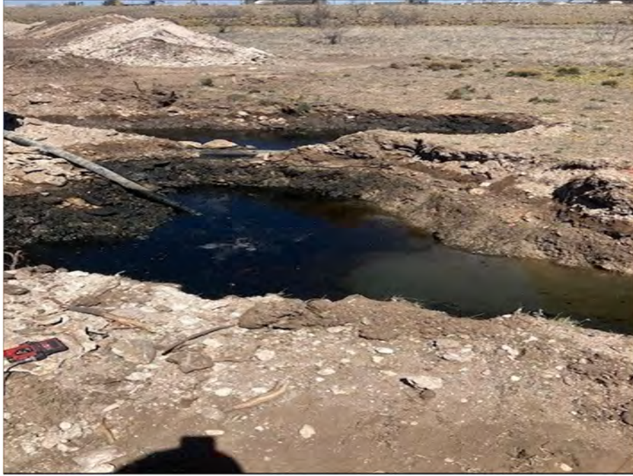
Pipeline Excavation Area:
