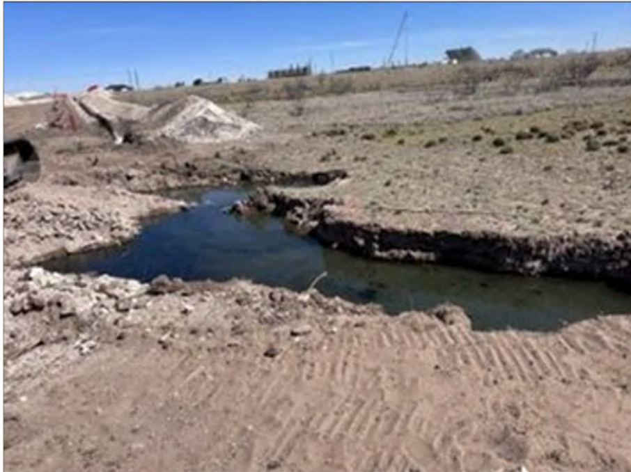
Pipeline Excavation Area:
