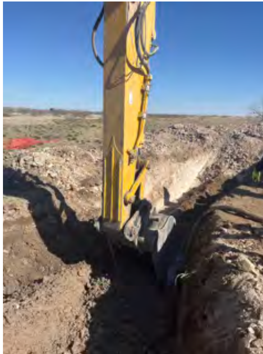
Pipeline Excavation Area:
