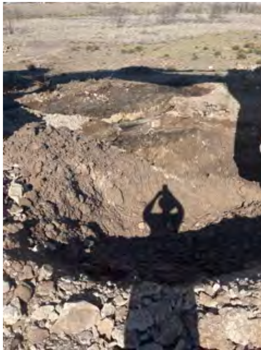
Pipeline Excavation Area:
