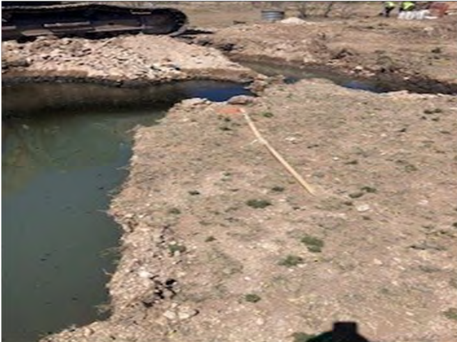
Pipeline Excavation Area:
