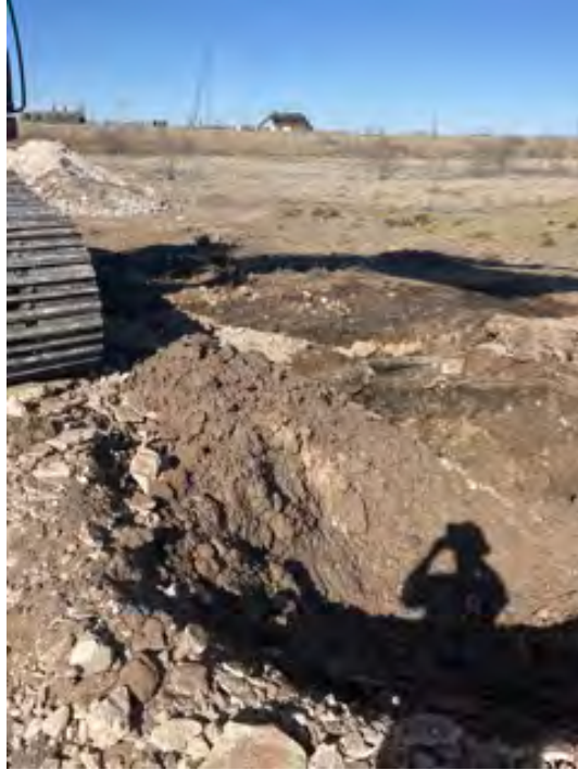
Pipeline Excavation Area:
