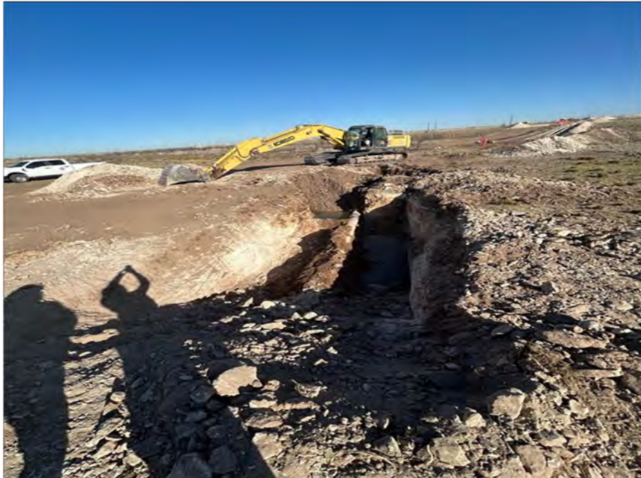
Pipeline Excavation Area:
