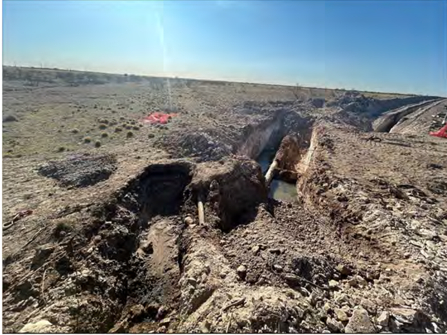
Pipeline Excavation Area:
