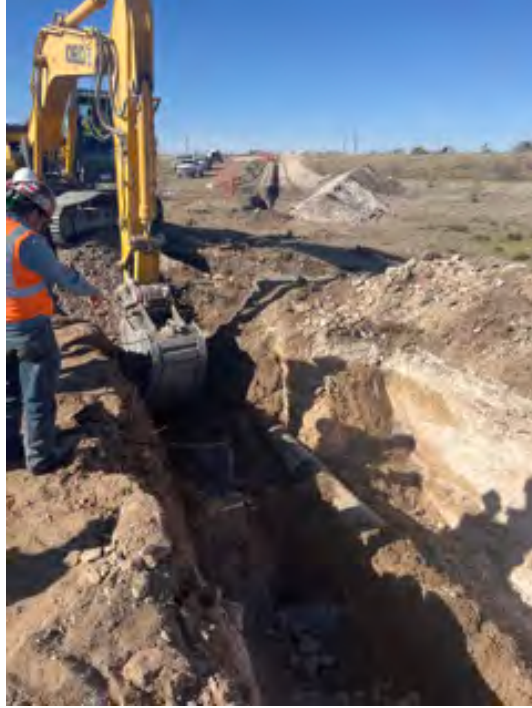
Pipeline Excavation Area:
