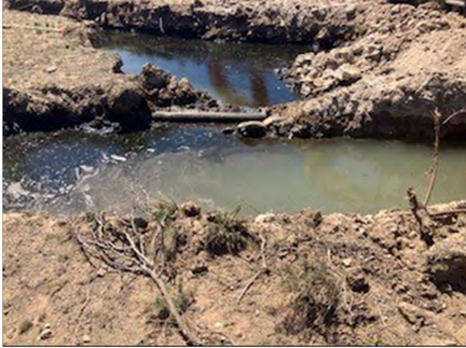
Pipeline Excavation Area:
