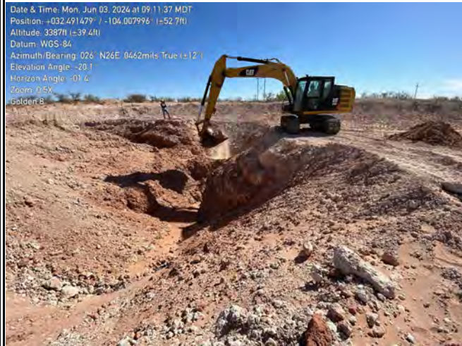
Photograph : 6 Date :6/3/2024 Description: Northern excavation View: Northeast
