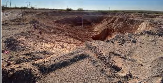
Photograph 1 Date :5/3/2024 Description: North portion of northern excavation View: East
