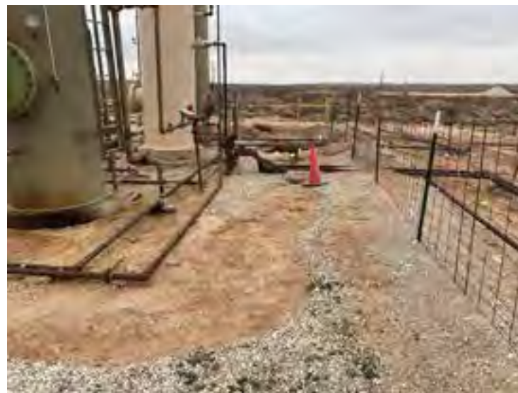
Photograph 4: View of equipment after hand shoveling activities.
