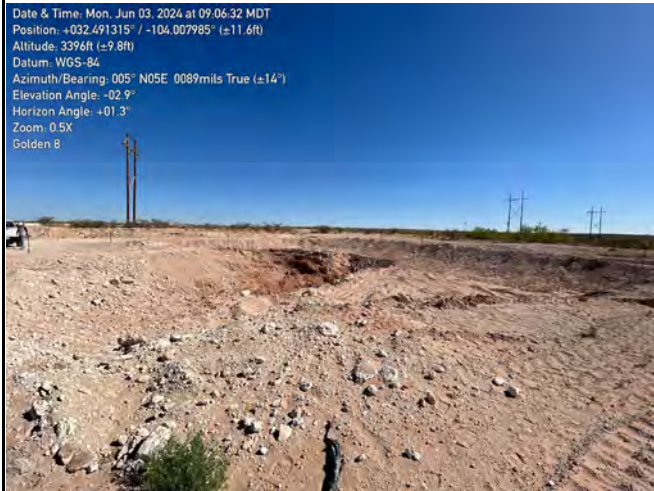
Photograph : 5 Date :6/3/2024 Description: Northern excavation View: North
