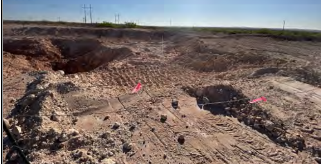
Photograph 3 Date :5/3/2024 Description: South portion of northern excavation View: Northeast
