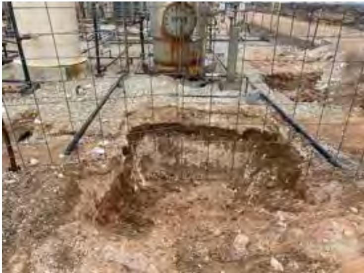
Photograph 7: View north of southern excavation activities.
