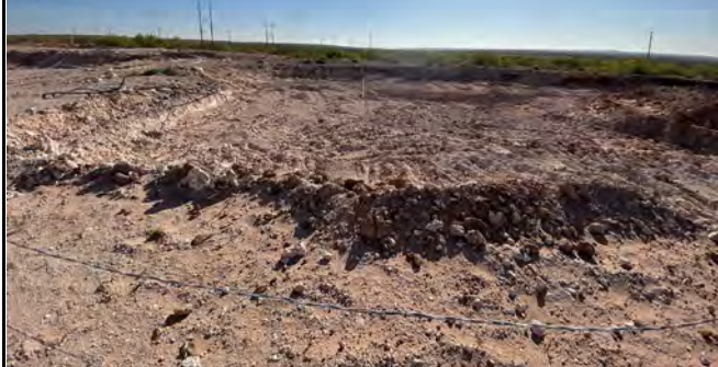
Photograph 4 Date :5/3/2024 Description: Southern excavation View: Northeast
