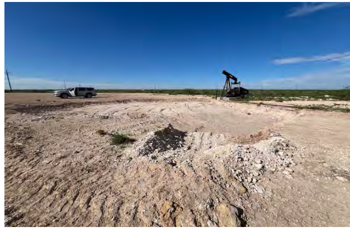
View to SW of well pad excavation (8/7/25).
