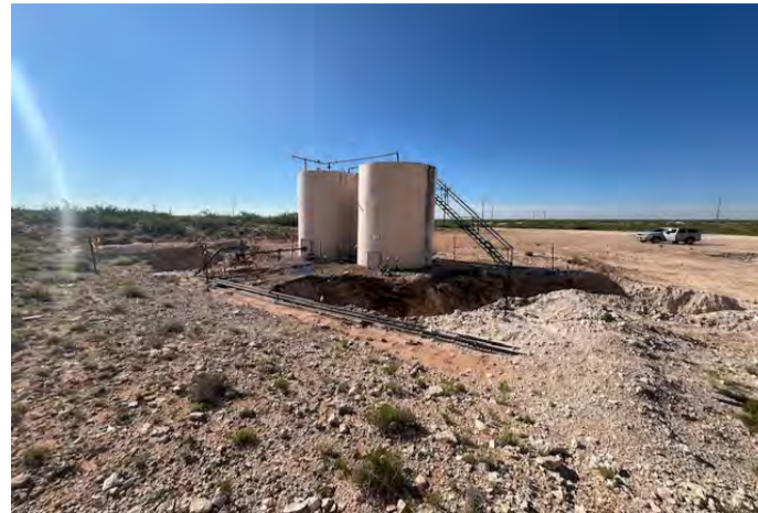
View to SE of TB excavations (8/7/25).
