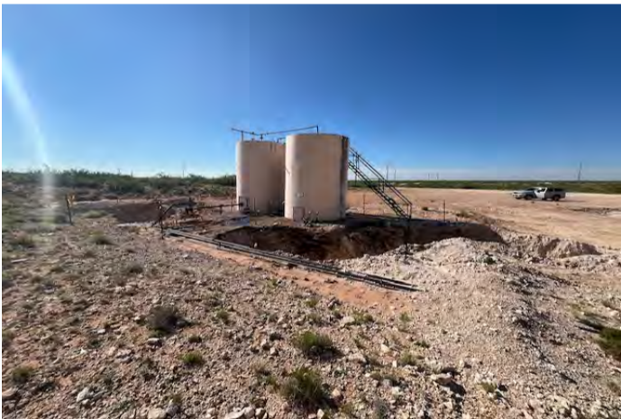
View to SE of TB excavations (8/7/25).
