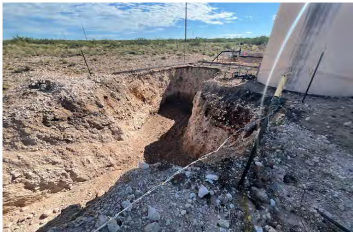
View to NW of W TB excavation (8/7/25).
