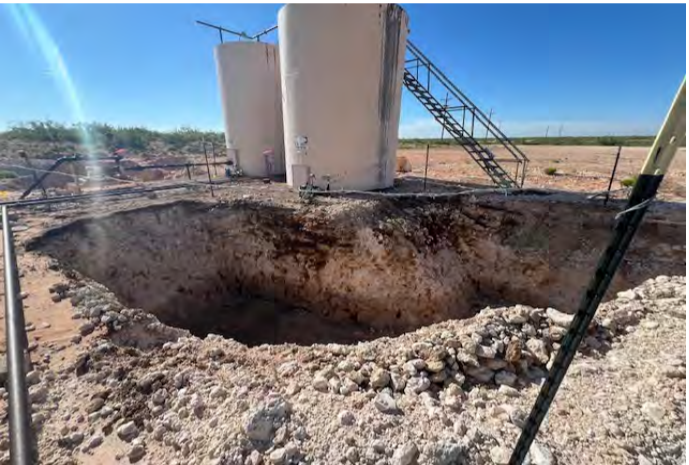
View to SE of W TB excavation (8/7/25).
