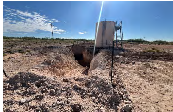
View to E of W TB excavation (8/7/25).
