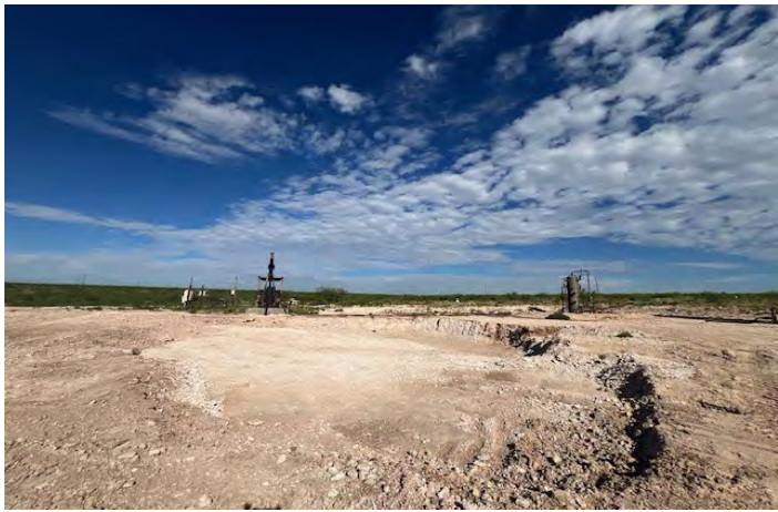
View to W of well pad excavation (8/7/25).
