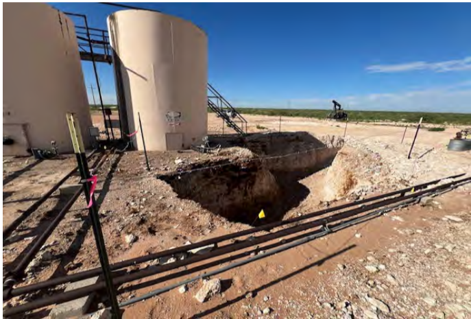
View to SW of E TB excavation (8/7/25).
