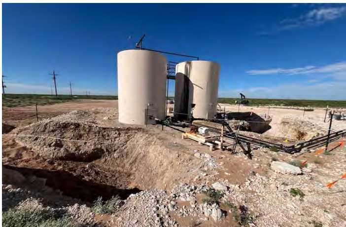
View to SW of TB excavations (8/7/25).
