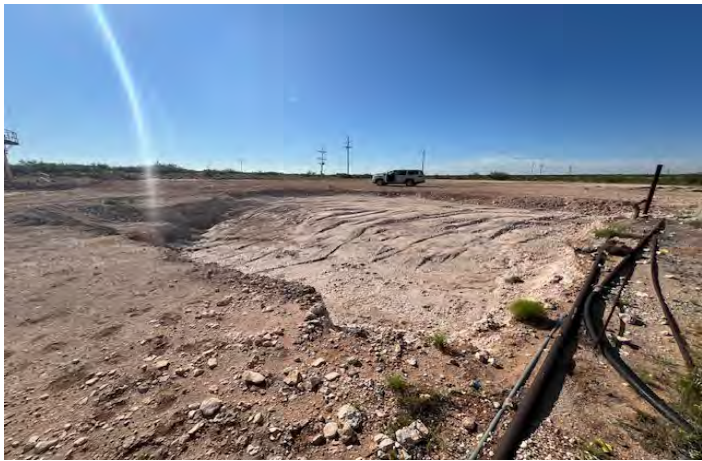
View to S of well pad excavation (8/7/25).
