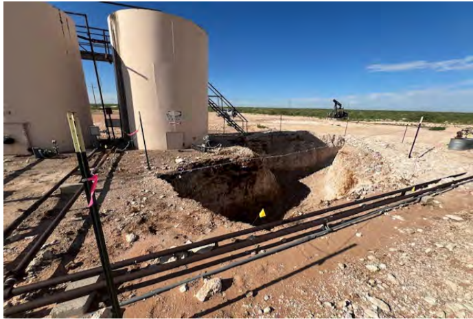
View to SW of E TB excavation (8/7/25).
