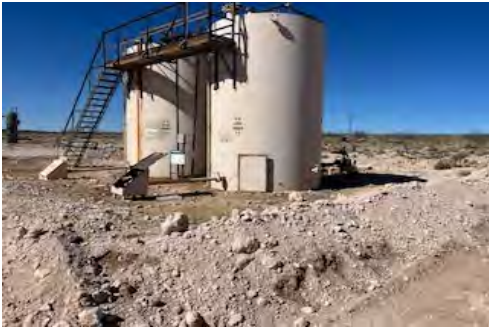
View to NW of backfilled excavations at battery (nSAP0225252743).
