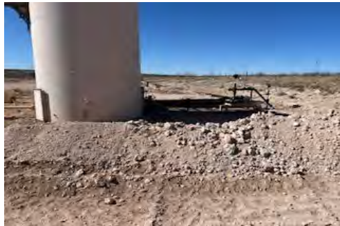
View to S of backfilled excavations at battery (nSAP0225252743).
