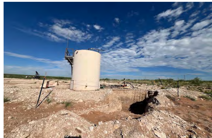
View to W of E TB excavation (8/7/25).
