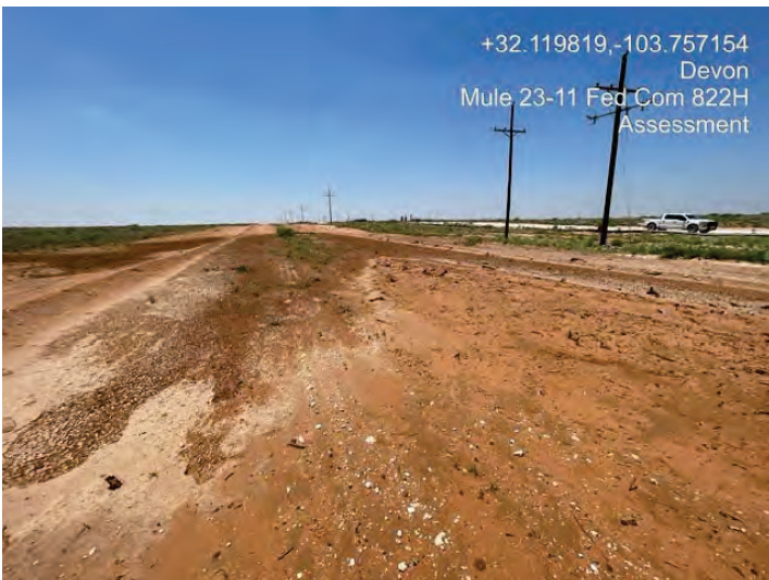
North side looking south
