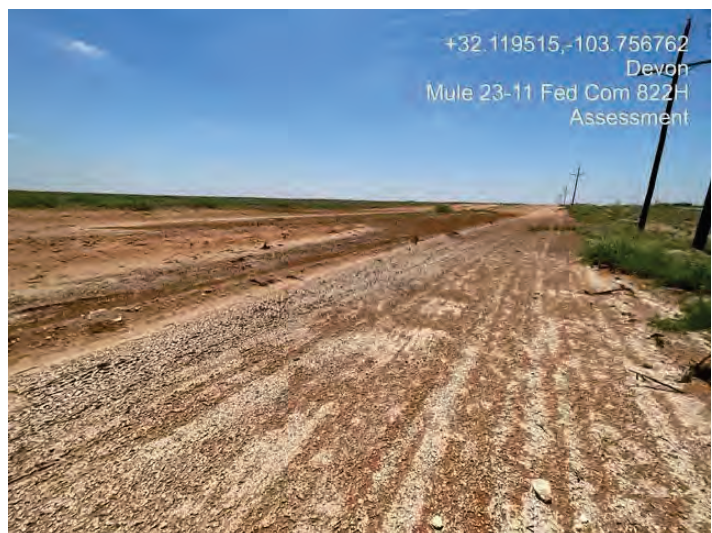
Northwest side looking southeast
