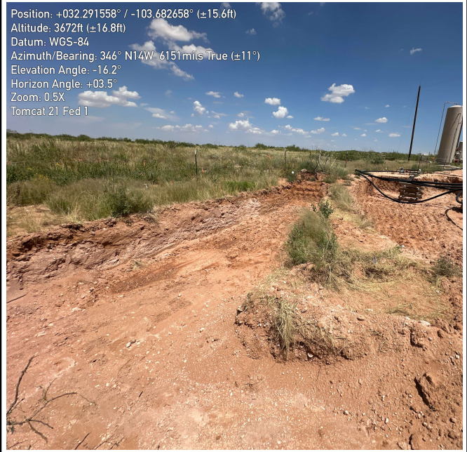
Photograph 2 Date: 07/29/2025 Description: Northwestern view of initial excavation area.
