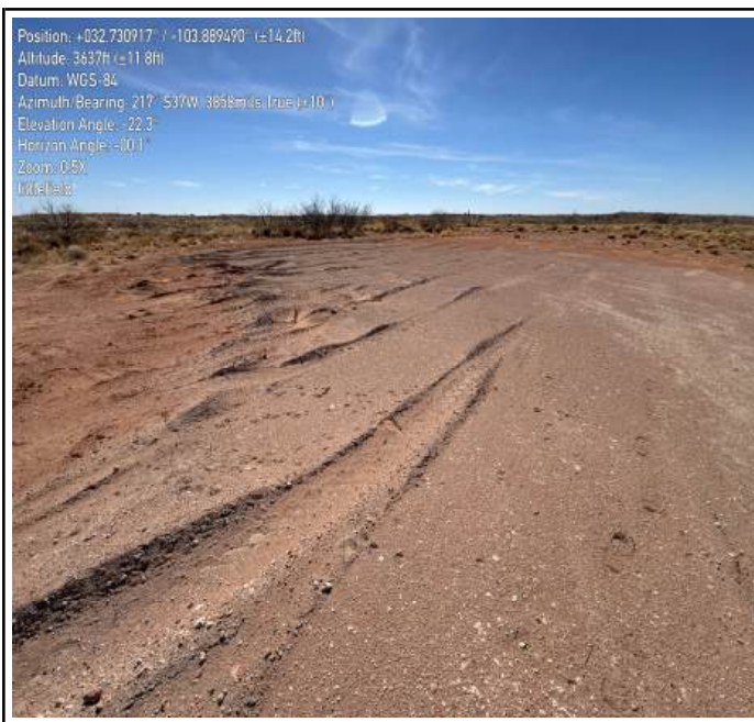
Photograph 7 Date: 02/27/2026 Description: Southwestern view of completed backfill activities.
