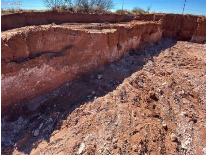
Photograph 3 Date: 01/15/2026 Description: Southwestern view of excavation confirmation activities.
