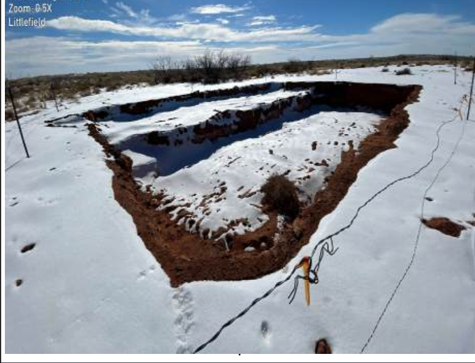
Photograph 4 Date: 01/28/2026 Description: Southwestern view of completed excavation.
