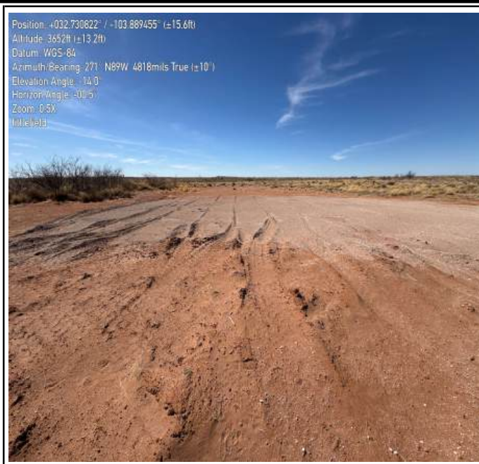
Photograph 6 Date: 02/27/2026 Description: Northwestern view of completed backfill activities.
