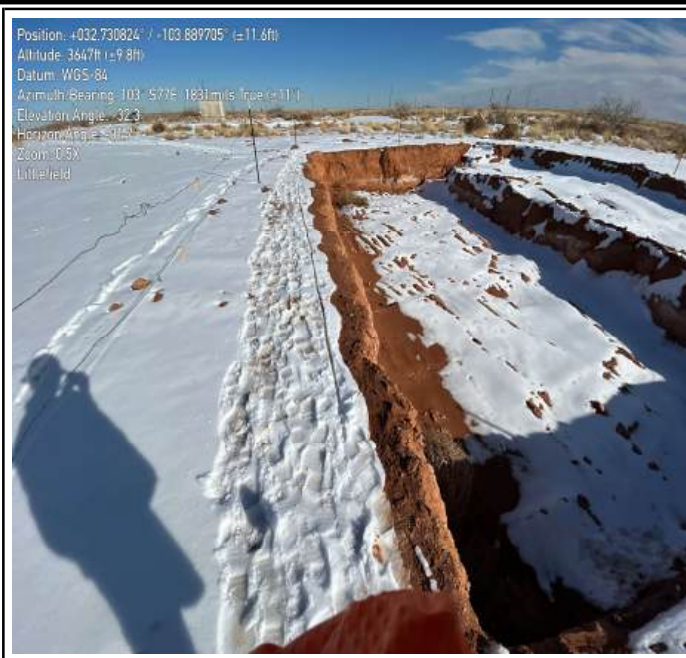
Photograph 5 Date: 01/28/2026 Description: Southeastern view of completed excavation.
