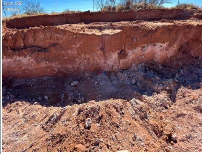
Photograph 2 Date: 01/15/2026 Description: Southwestern view of excavation confirmation activities.
