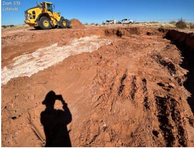
Photograph 1 Date: 01/15/2026 Description: Northeastern view of excavation confirmation activities.
