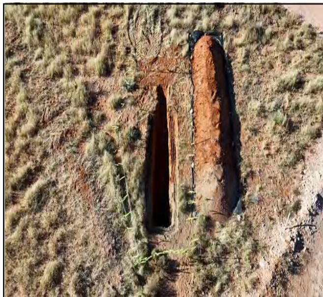
Photo taken during excavation process.
