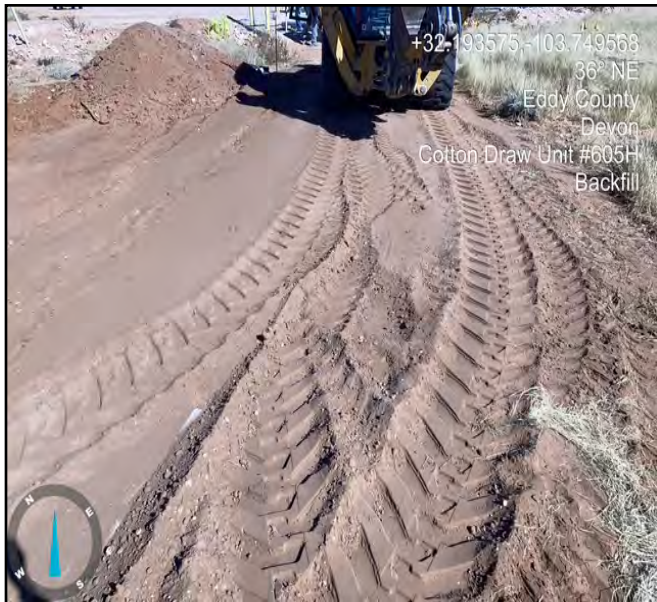
Photo taken post backfill.
