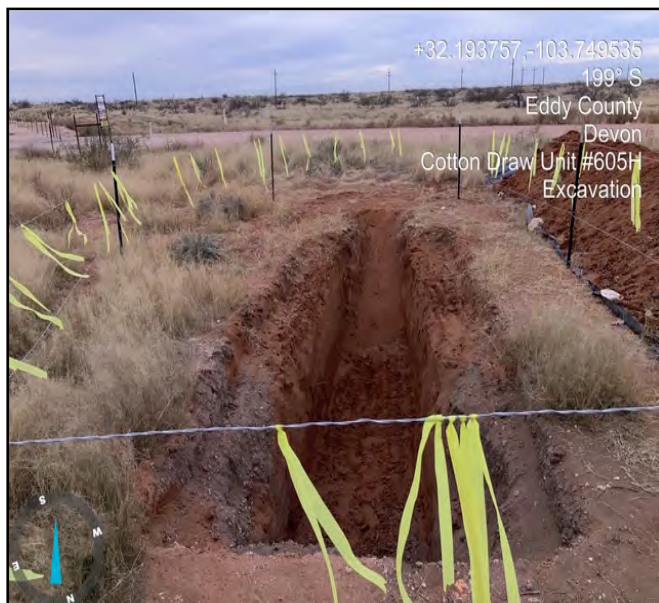
Photo taken during excavation process facing south.
