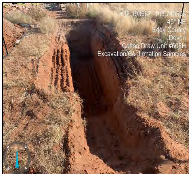
Photo taken during excavation process facing northeast.
