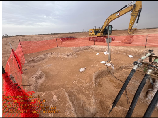
2ft and 3ft bgs excavation.
