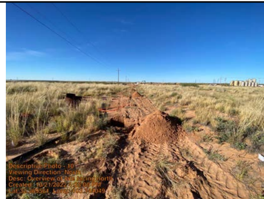
Overview of site facing north
