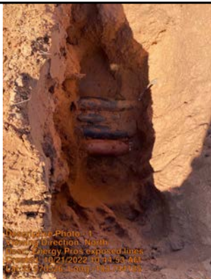
Energy Pros exposed lines
