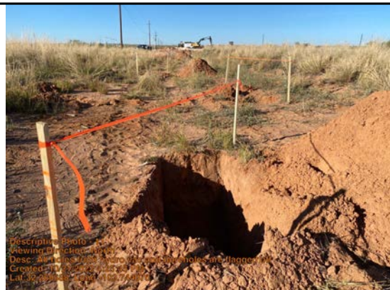
All holes from hydro vac and boreholes are flagged off
