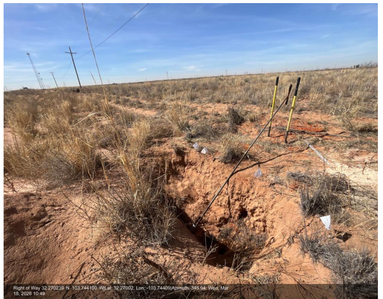
Right of Way 32.270239 N 103.744100 W|Lat: 32.27002, Lon: -103.74409|Azimuth: 345.94, Wed, Mar 18, 2026 10:49
