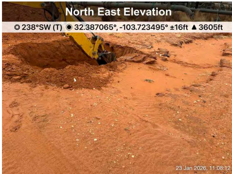
Photographs 30 (01/23/2026): Photograph of the secondary release area, viewing northeast.
