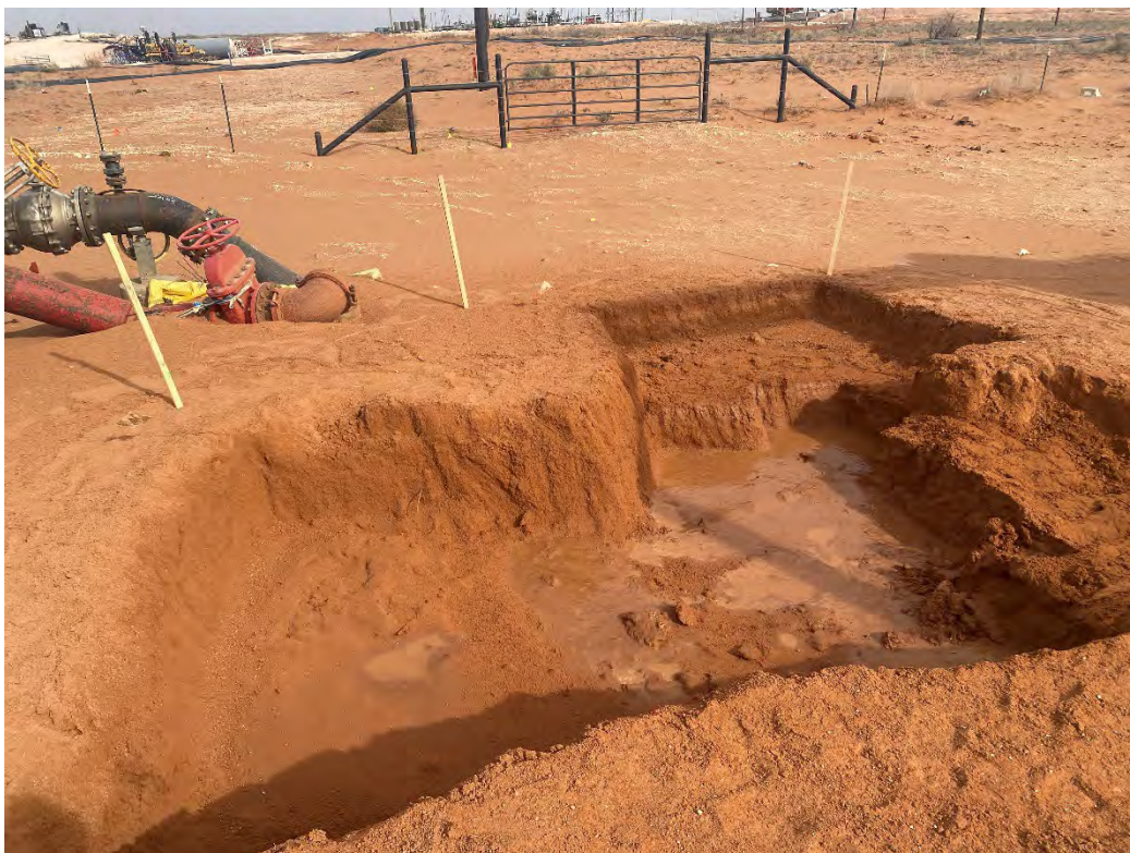
Photograph 16 (03/07/2025): Sample locations CS-52 through CS-54 at 2'bgs; facing northeast.
