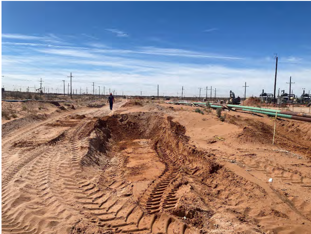
Photograph 21 (03/24/2025): Additional excavation at sample location CS-48 to 4' bgs; facing south.
