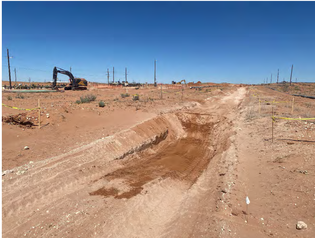
Photograph 23 (03/25/2025): Additional excavation at sample location CS-89 to 4' bgs; facing southeast.
