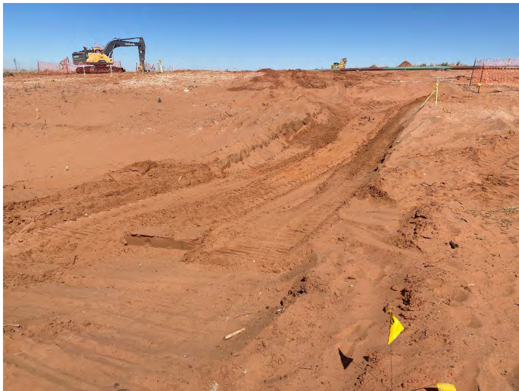
Photograph 24 (03/25/2025): Additional excavation at sample location CS-20 and CS-22 to 4' bgs; facing northwest.
