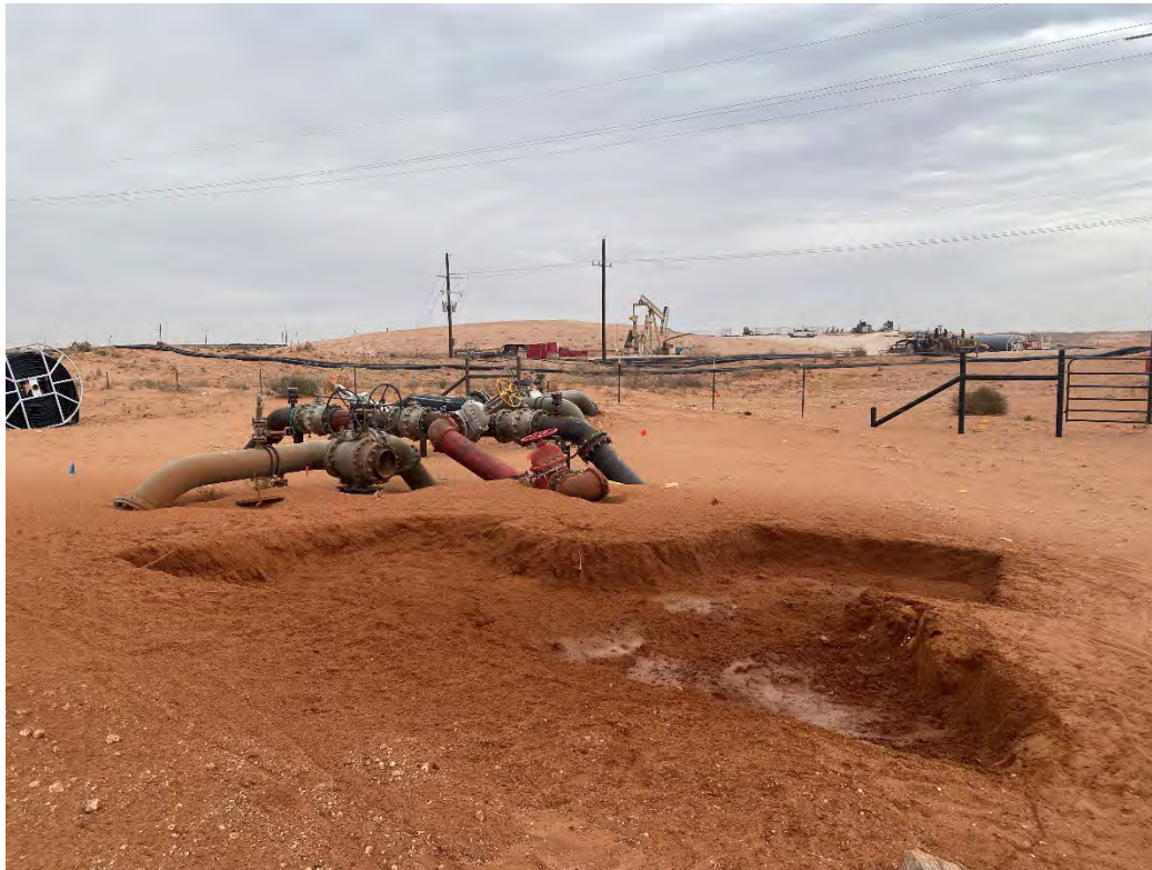
Photograph 15 (03/07/2025): Sample locations CS-52 through CS-54 at 1'bgs; facing northeast.
