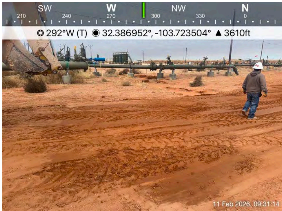
Photographs 32 (02/11/2026): Photograph of the secondary release area backfilled, viewing west.
