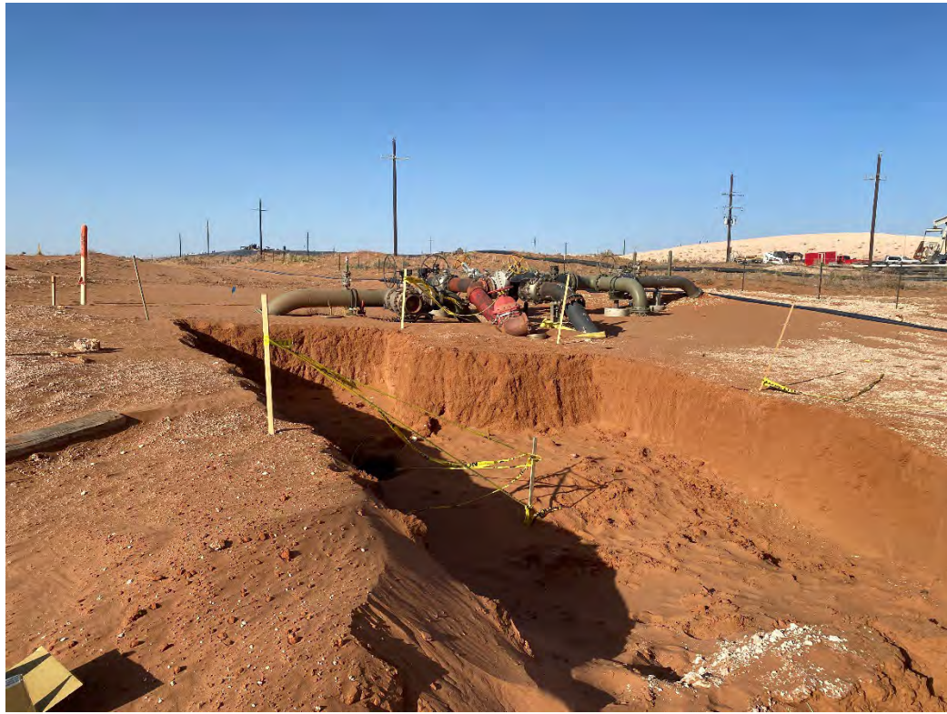
Photograph 17 (03/12/2025): Sample locations CS-50 and CS-52 through CS-54 at 4' bgs; facing northeast.
