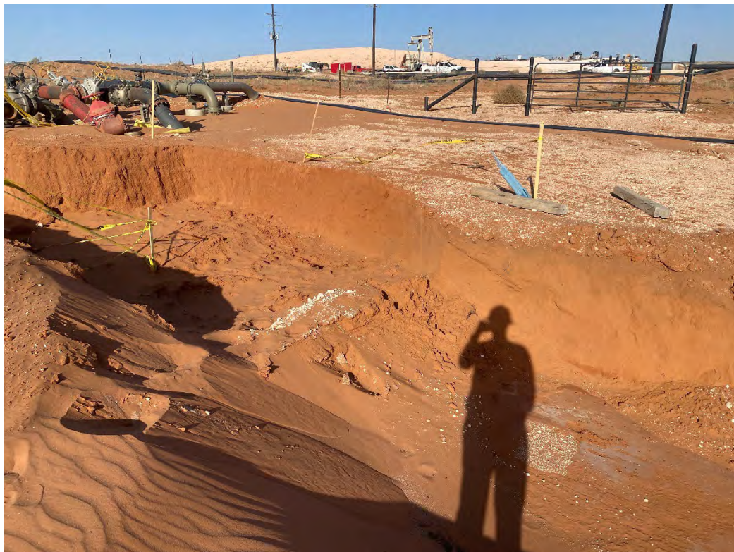
Photograph 18 (03/12/2025): Sample locations CS-50 and CS-52 through CS-54 at 4' bgs; facing northeast.
