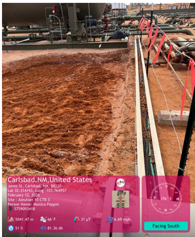
Wall in middle of excavation 0-1.5'.
