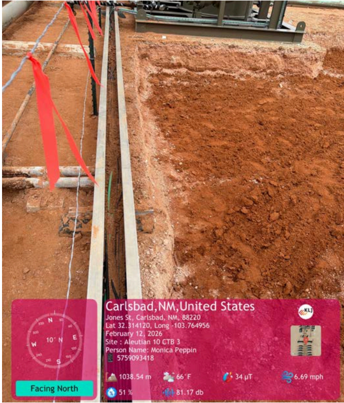
Middle area of excavation.
