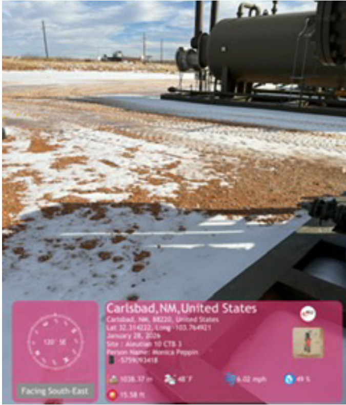
1.5' excavation from northwest corner.
