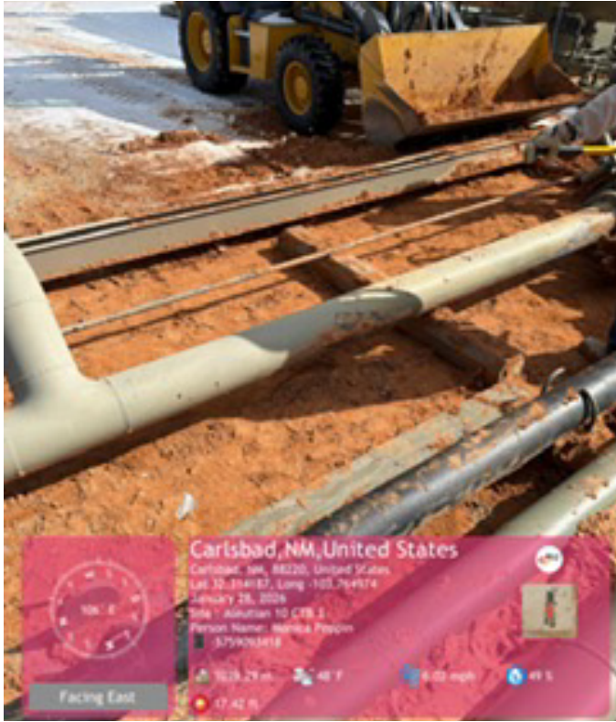
1.5' excavation from northwest corner.
