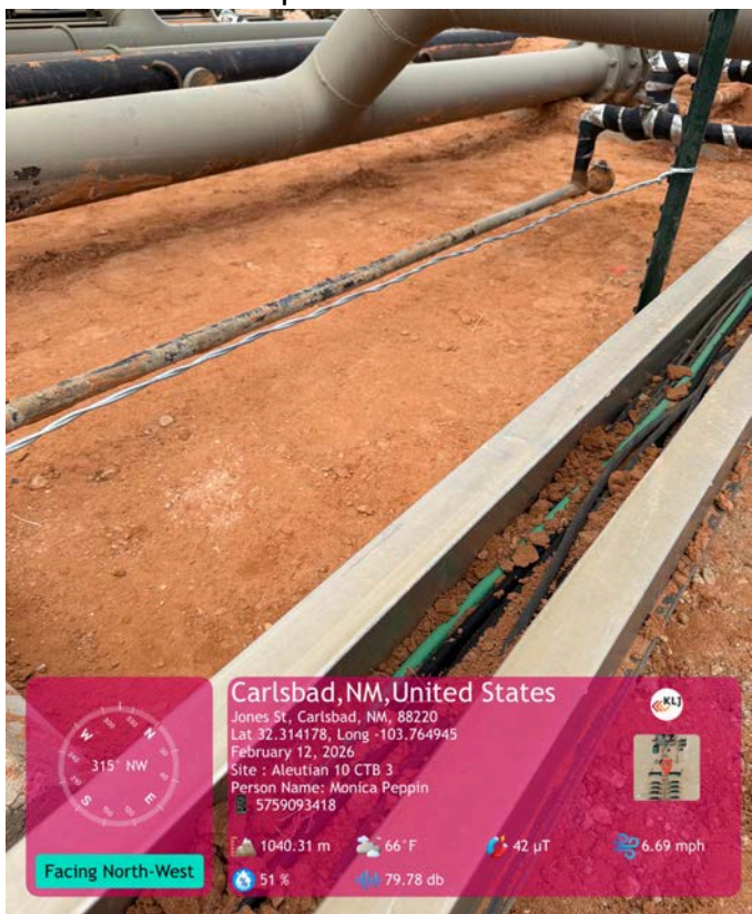
Hand excavated area under piping at start of deeper excavation.
