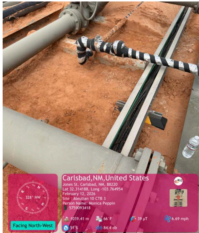
Hand excavation area under piping.
