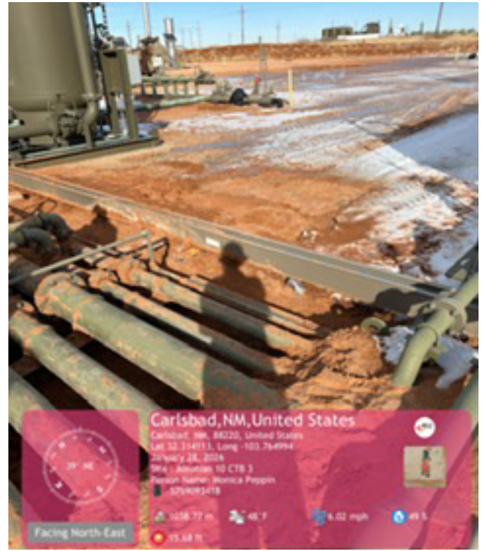
1.5' excavation from southwest corner.
