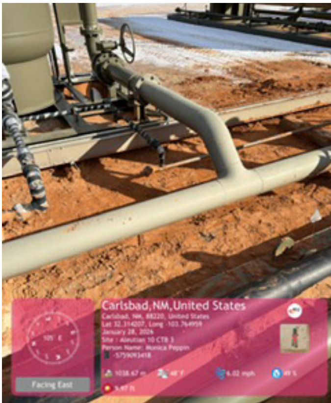
East wall area of 1.5' excavation.
