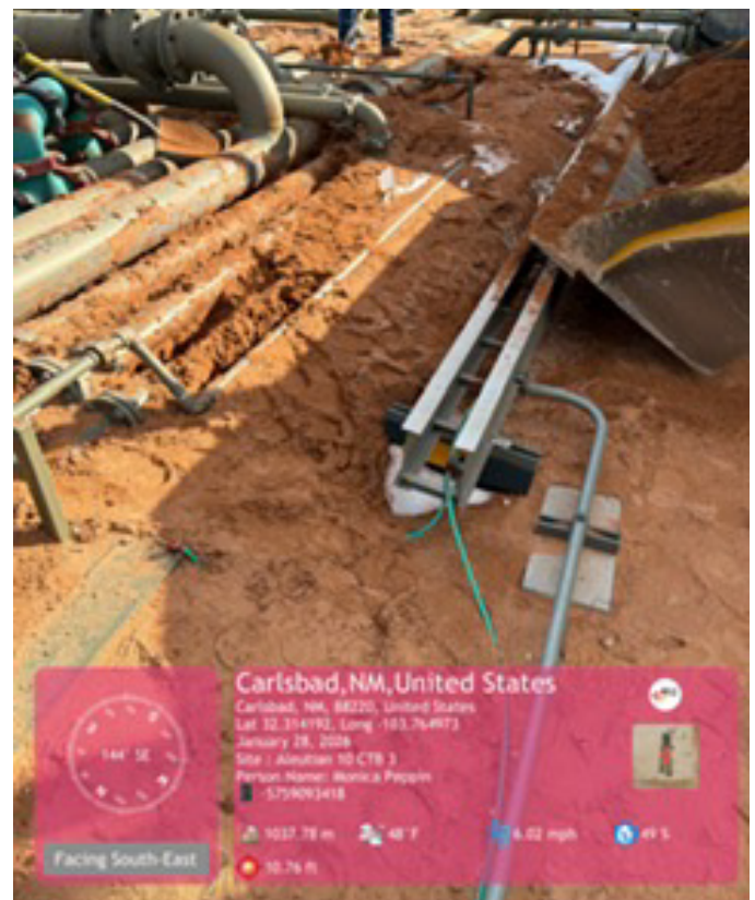
0.5' excavation under piping on west end.
