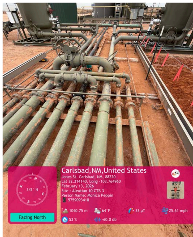
North view of hand excavated area.
