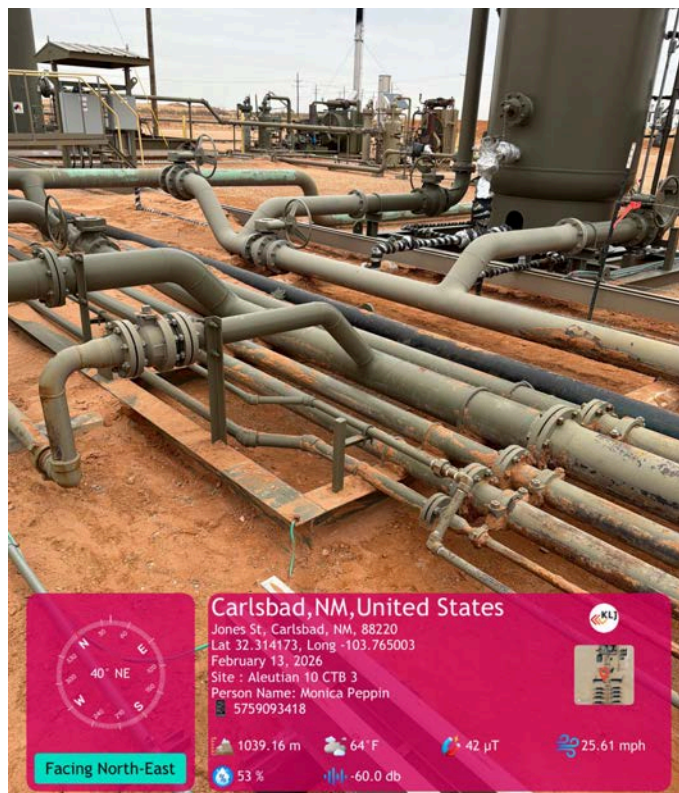
Equipment and piping where addtl. excavation occurred.
