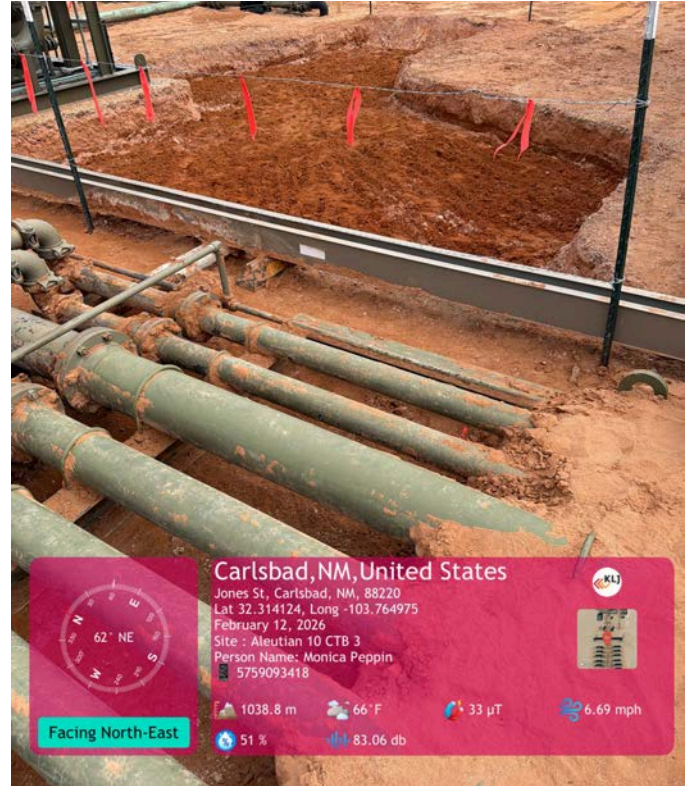
Hand excavation area and fencing.
