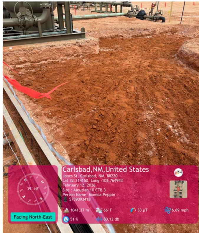
1.5' excavation from southwest corner.
