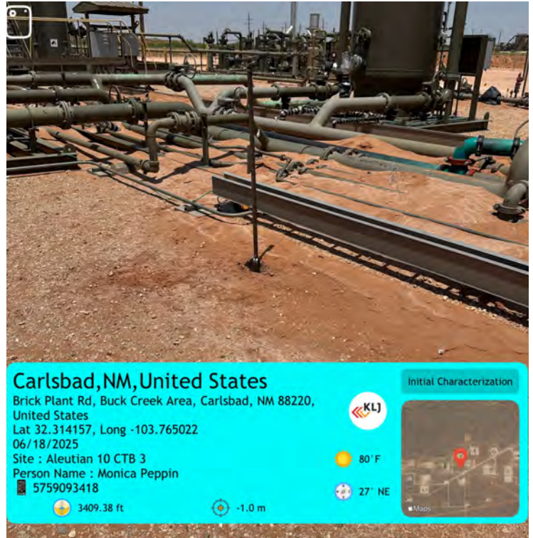
BH05 on west side of equipment.
