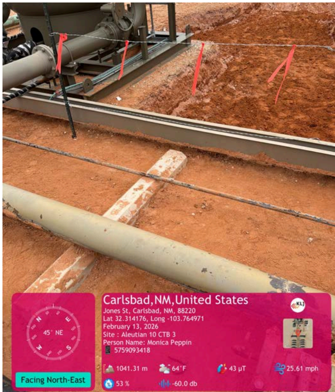
Northwest corner of 1.5' excavation.
