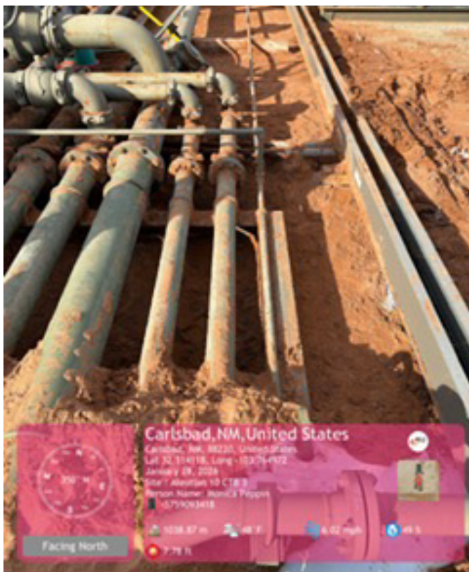
East wall area of 1.5' excavation.
