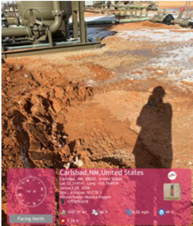
1.5' excavation from northwest corner.
