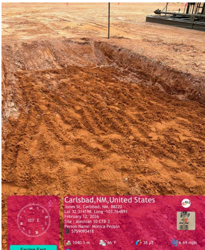
East wall area of 1.5' excavation.
