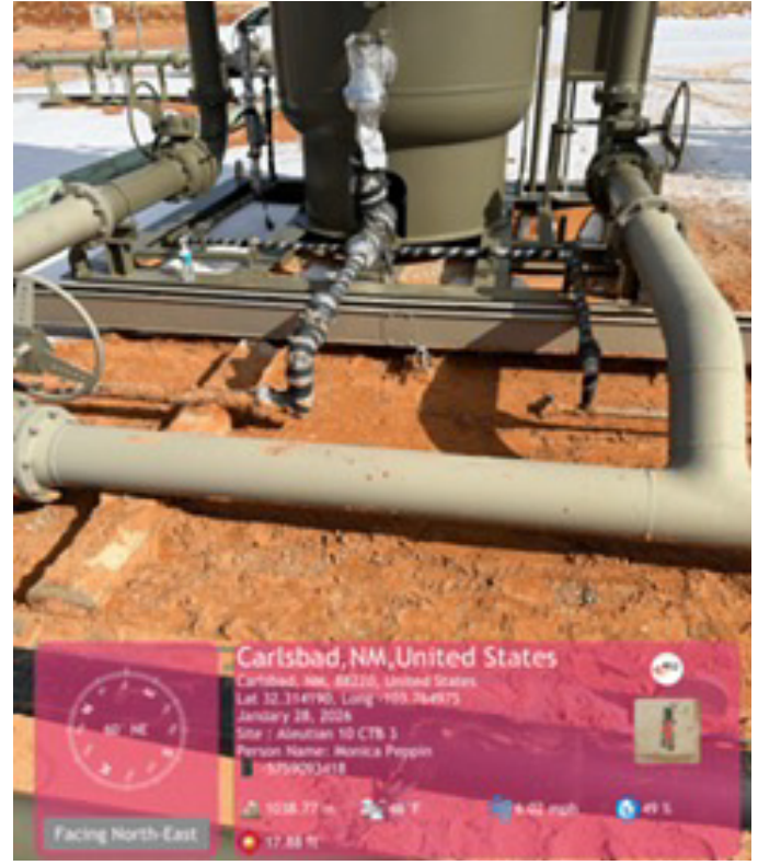
1.5' excavation from southwest corner.
