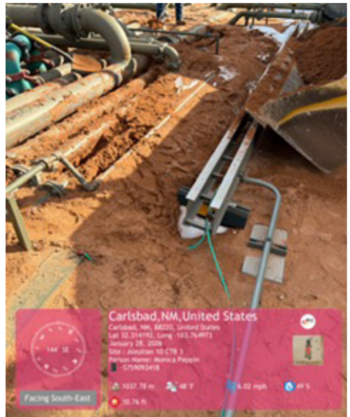
0.5' excavation under piping on west end.
