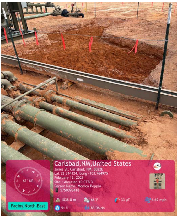
Hand excavated area under piping and 1.5' excavation.
