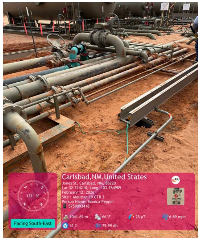
Hand excavated area.
