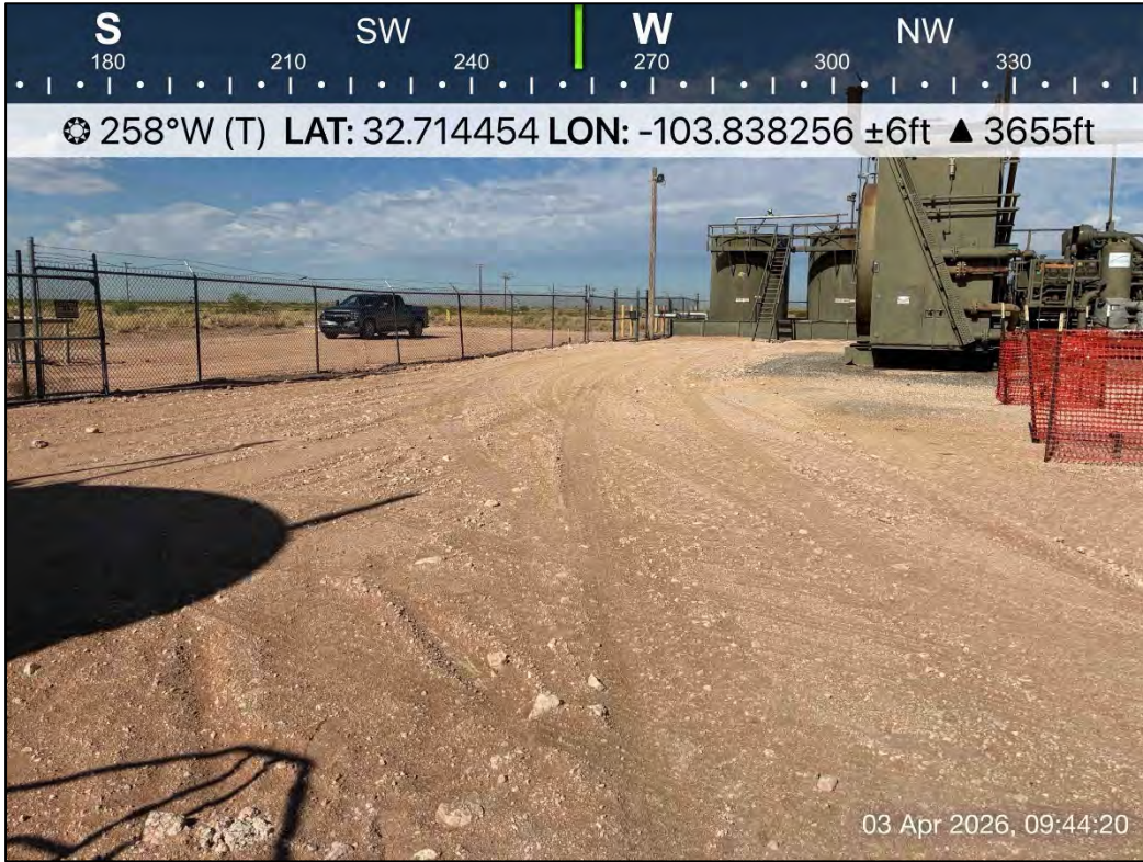
PHOTO 15: Southeastern view following restoration activities. 4/3/2026
