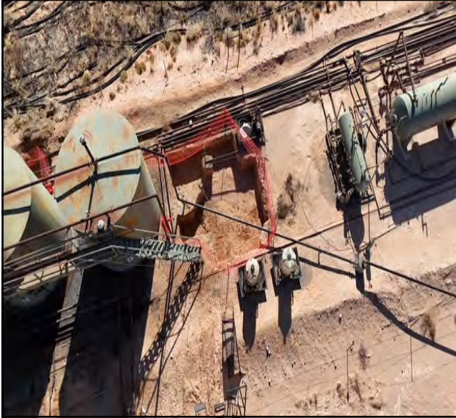
Aerial photos taken during excavation.
