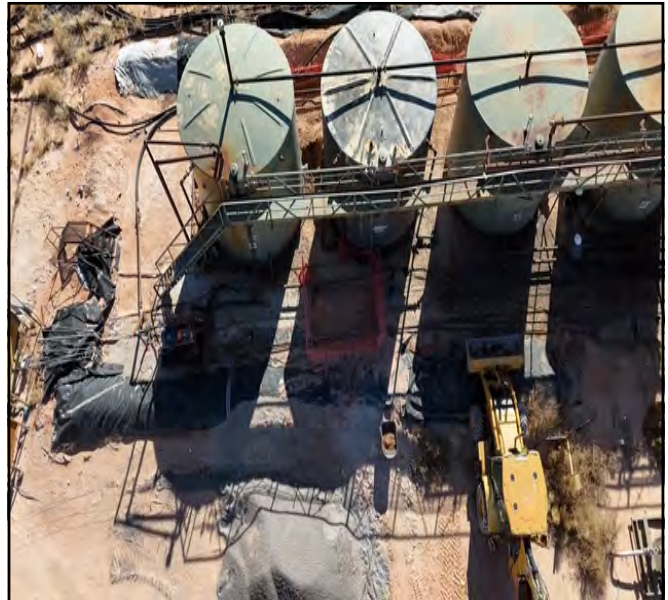
Aerial photos taken during excavation.
