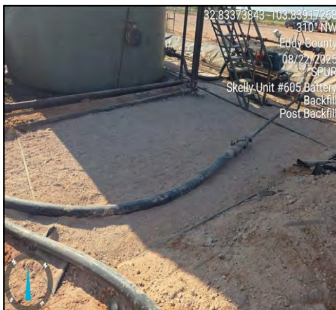
Photo taken post excavation facing northwest.
