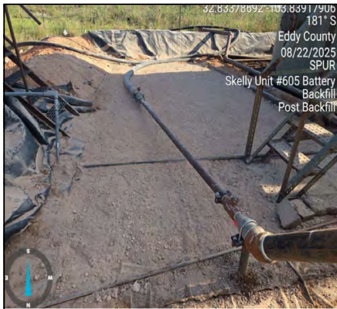
Photo taken post excavation facing south.
