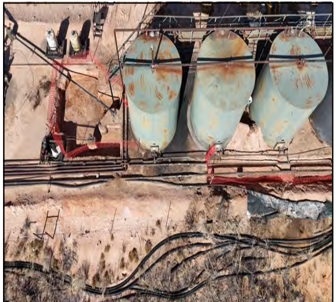
Aerial photos taken during excavation.
