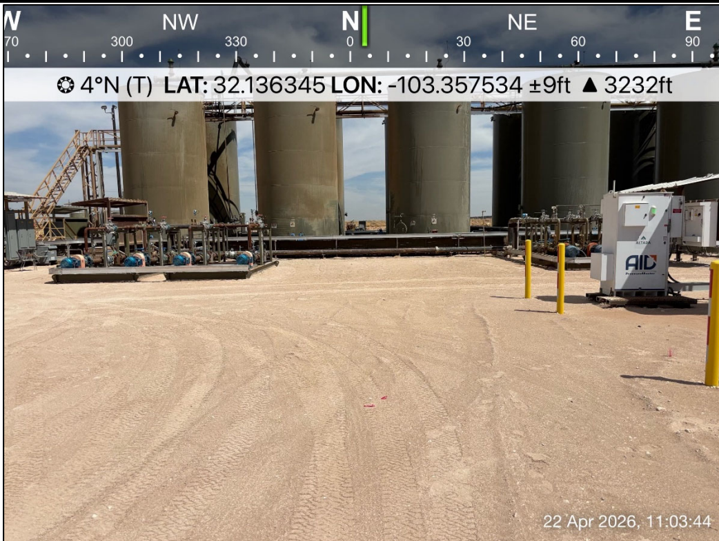
PHOTO 30: Northern view following restoration activities. 4/22/2026
