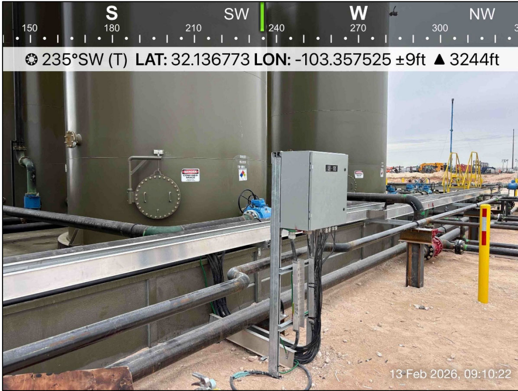
PHOTO 7: Southwestern view outside of containment during liner inspection activities. 2/13/2026
