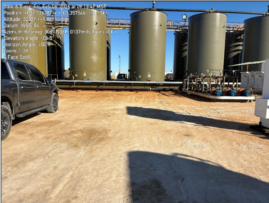
PHOTO 2: Northeastern view during initial site assessment activities. 2/6/2026
