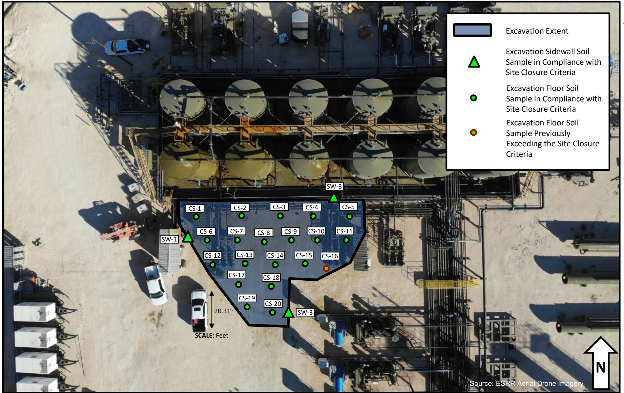
Figure 3 – Excavation Soil Sample Locations
