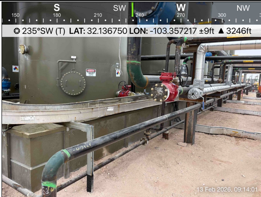
PHOTO 8: Southwestern view outside of containment during liner inspection activities. 2/13/2026
