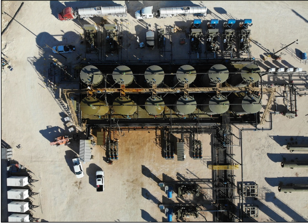
PHOTO 1: Northern aerial view during initial site assessment activities. 2/6/2026
