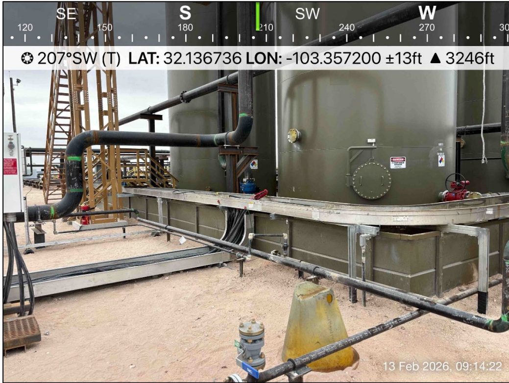
PHOTO 9: Southwestern view outside of containment during liner inspection activities. 2/13/2026
