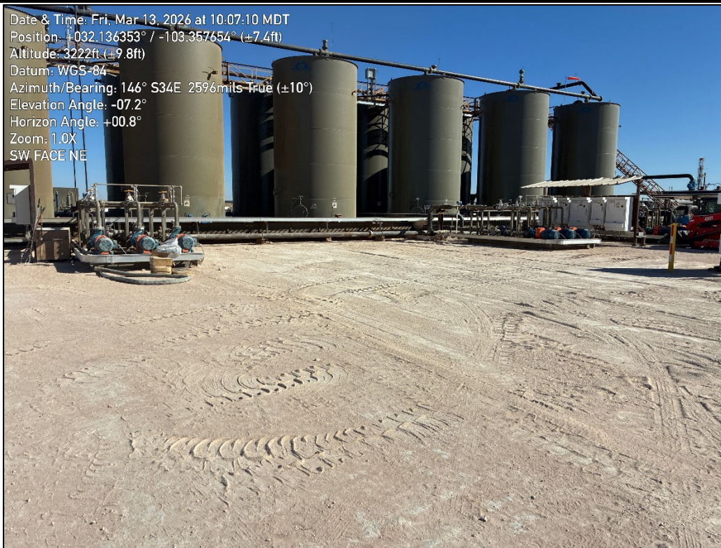
PHOTO 28: Southeastern view following initial excavation activities. 3/13/2026
