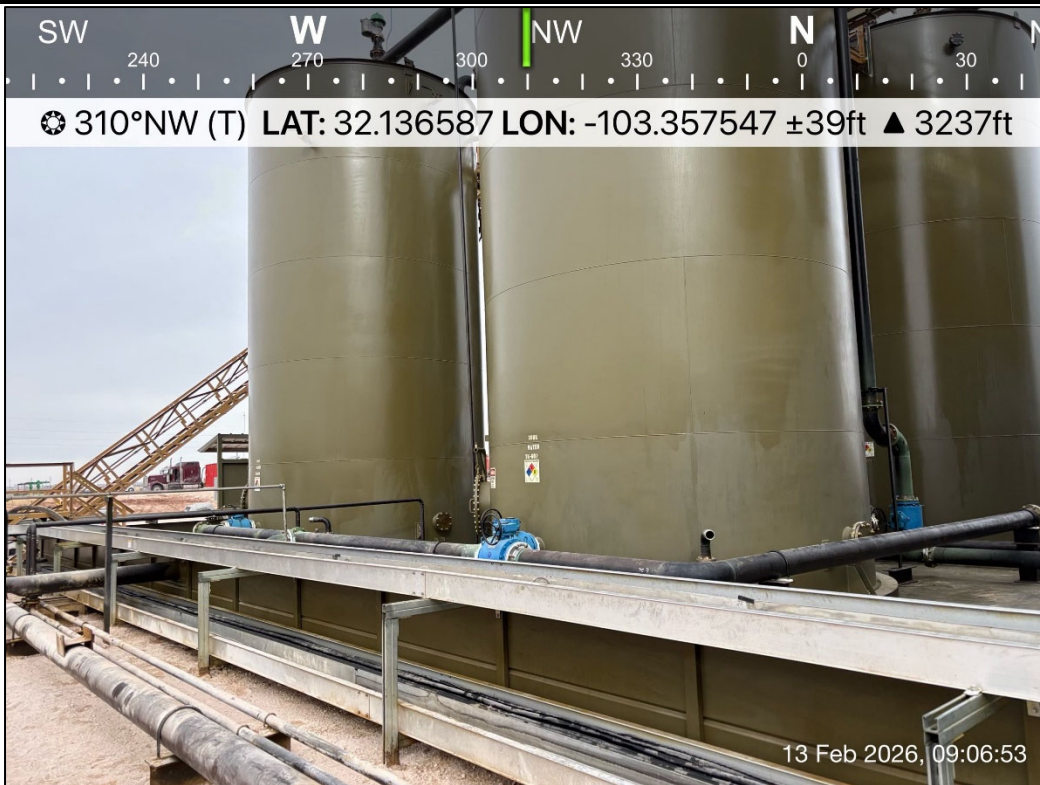
PHOTO 4: Northwestern view outside of containment during liner inspection activities. 2/13/2026
