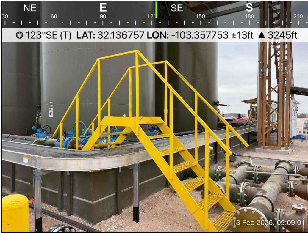
PHOTO 5: Southeastern view outside of containment during liner inspection activities. 2/13/2026
