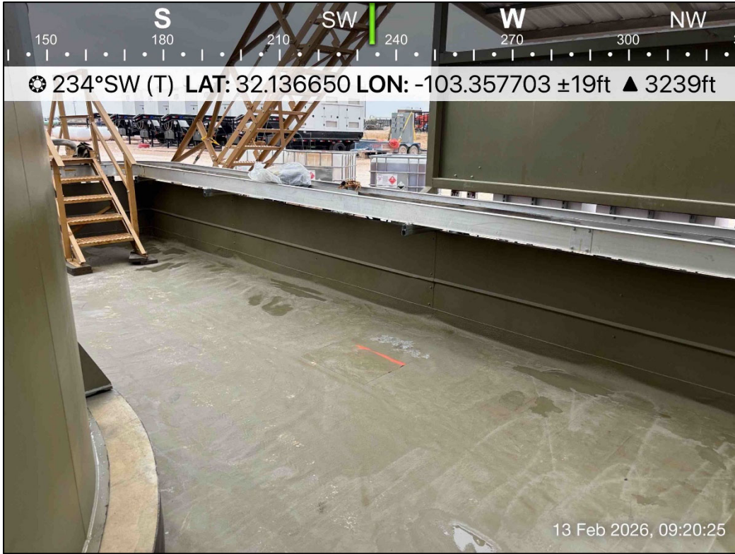
PHOTO 15: Southwestern view during liner inspection activities. 2/13/2026
