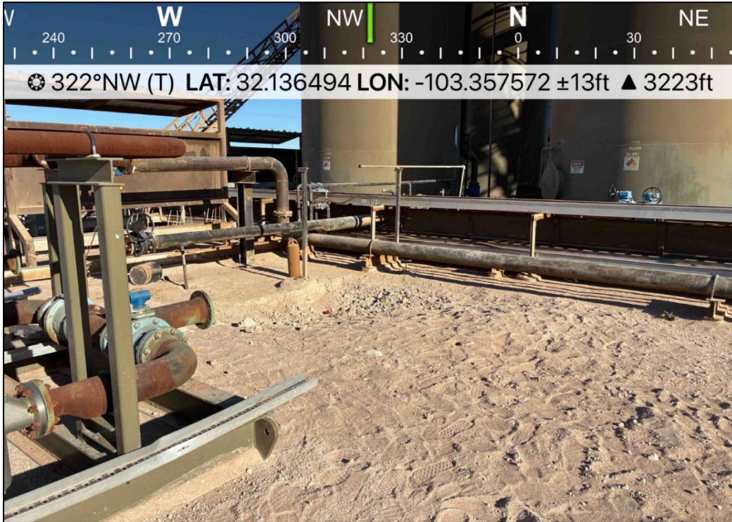
PHOTO 29: Northwestern view following initial excavation activities. 3/13/2026
