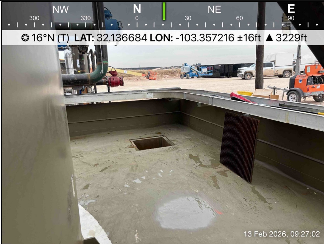
PHOTO 19: Northeastern view during liner inspection activities. 2/13/2026
