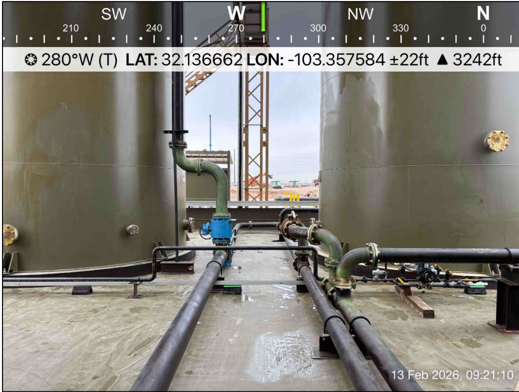
PHOTO 17: Northwestern view during liner inspection activities. 2/13/2026
