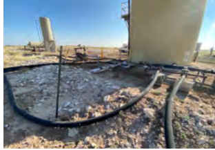
Soil staining at water tank (9/2/21).
