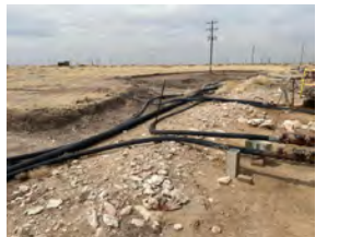
Excavated area to west of well pad (4/19/22).
