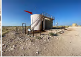
View of staining at Tank Battery (9/2/21).
