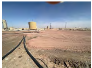
View to E of backfilled excavation (4/4/23).
