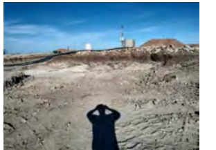
Excavated area to southwest of well pad (3/6/23).
