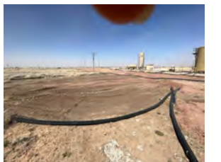
View to N of backfilled excavation (4/4/23).
