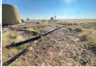
Barren area to south of Tank Battery (9/2/21).
