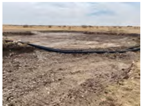
Excavated area to southwest of well pad (4/19/22).
