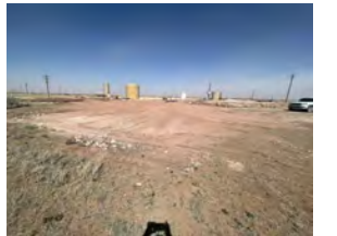
View to east of backfilled excavation (4/4/23).
