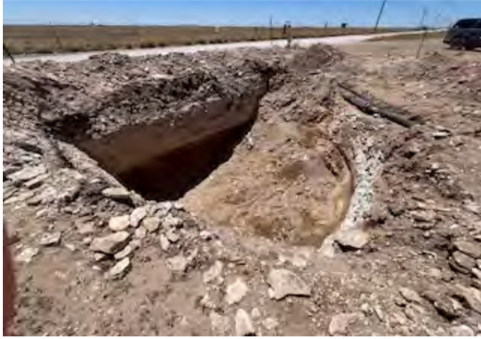
View to SW of W excavation.
