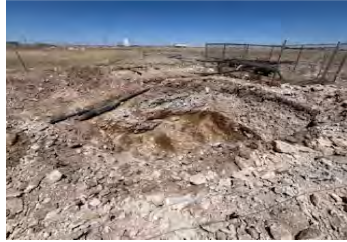
View to NE of W excavation.
