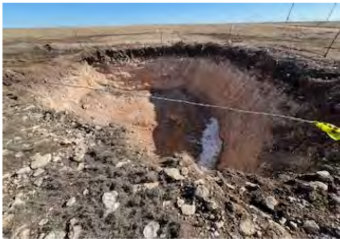
View to E of E excavation.
