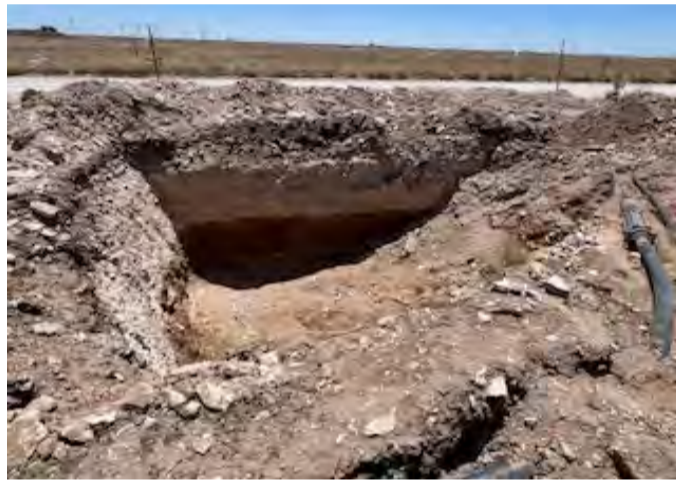
View to S of W excavation.
