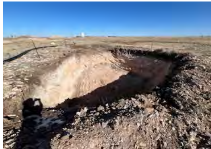
View to N of E excavation.
