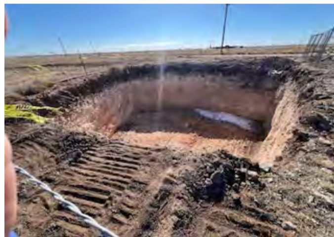
View to S of E excavation.
