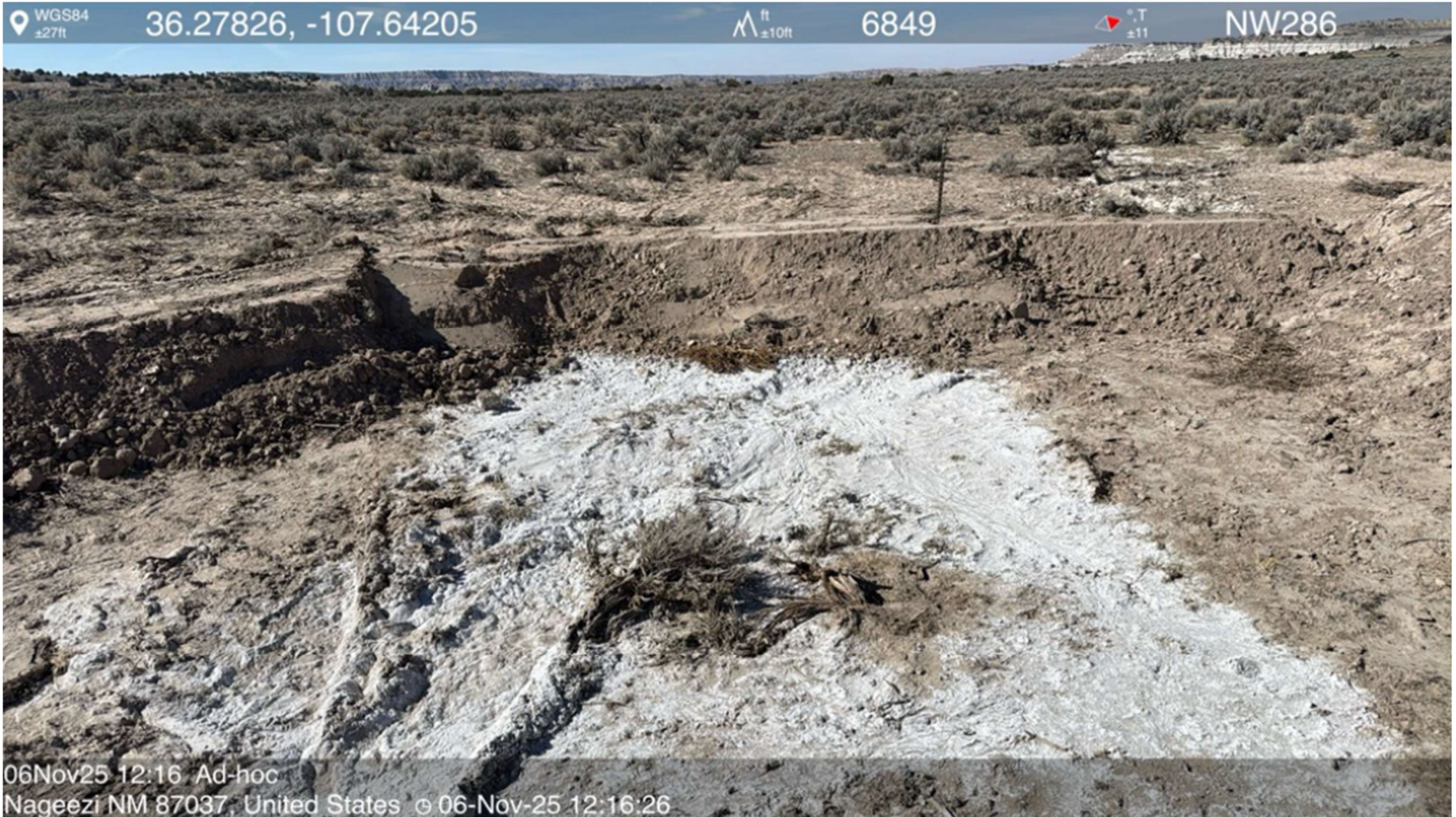
Photo #4 Earthen berm to contain release on-pad.
