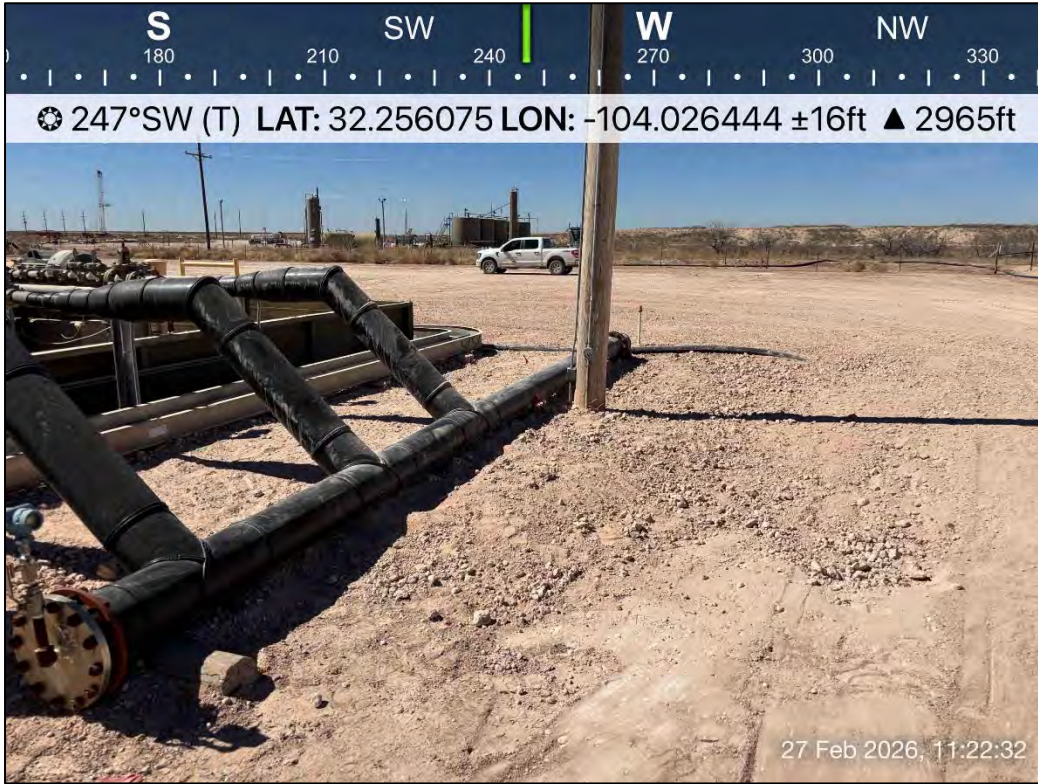
PHOTO 17: Southwestern view following restoration activities. 2/27/2026
