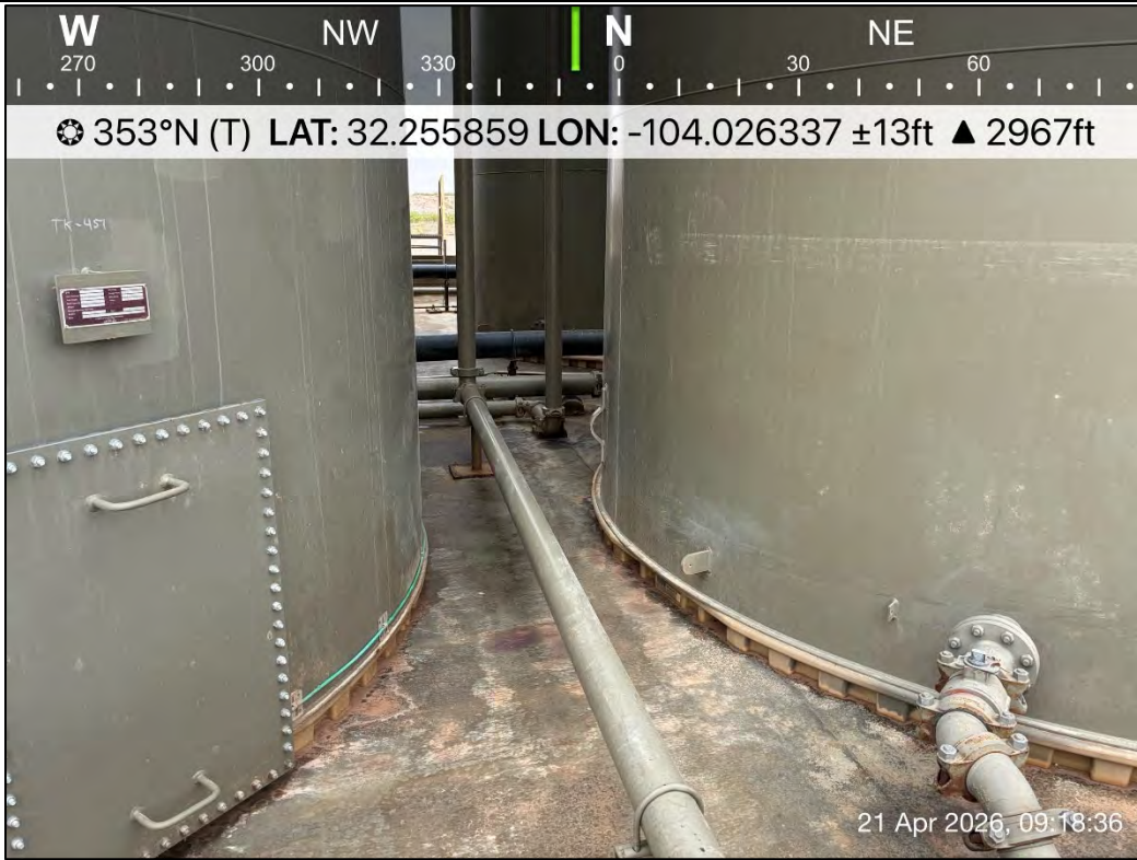
PHOTO 29: Northern view during liner inspection activities. 4/21/2026
