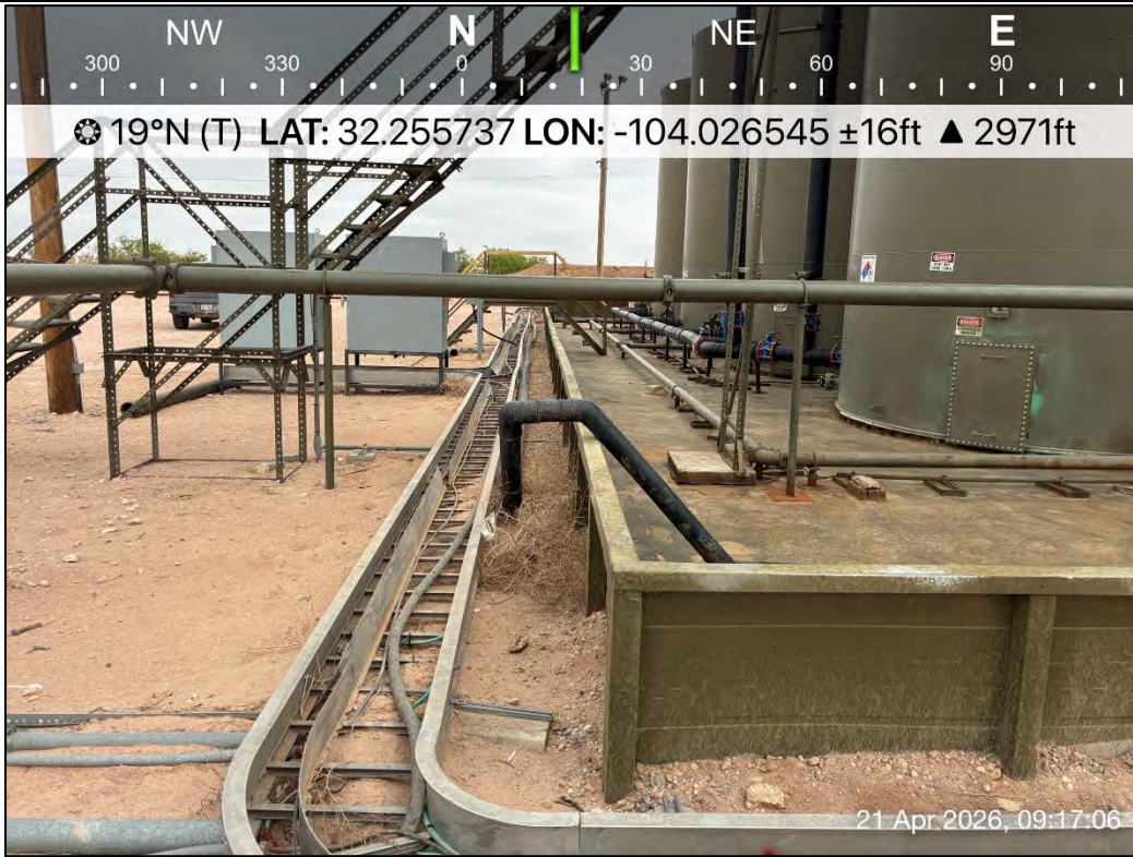
PHOTO 19: Northeastern view outside of containment during liner inspection activities. 4/21/2026
