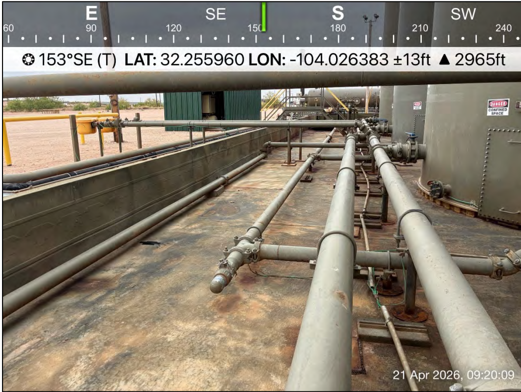
PHOTO 31: Southeastern view during liner inspection activities. 4/21/2026
