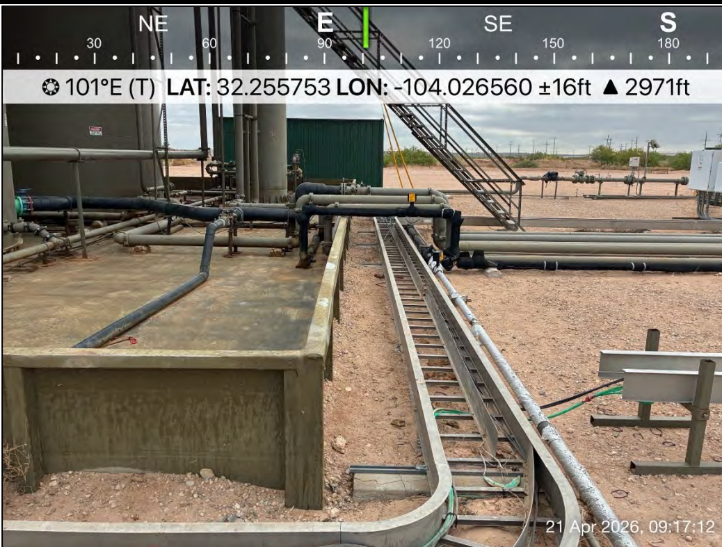
PHOTO 20: Southeastern view outside of containment during liner inspection activities. 4/21/2026
