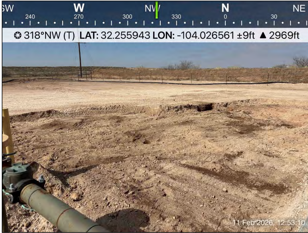
PHOTO 13: Northwestern view of excavation extent. 2/11/2026
