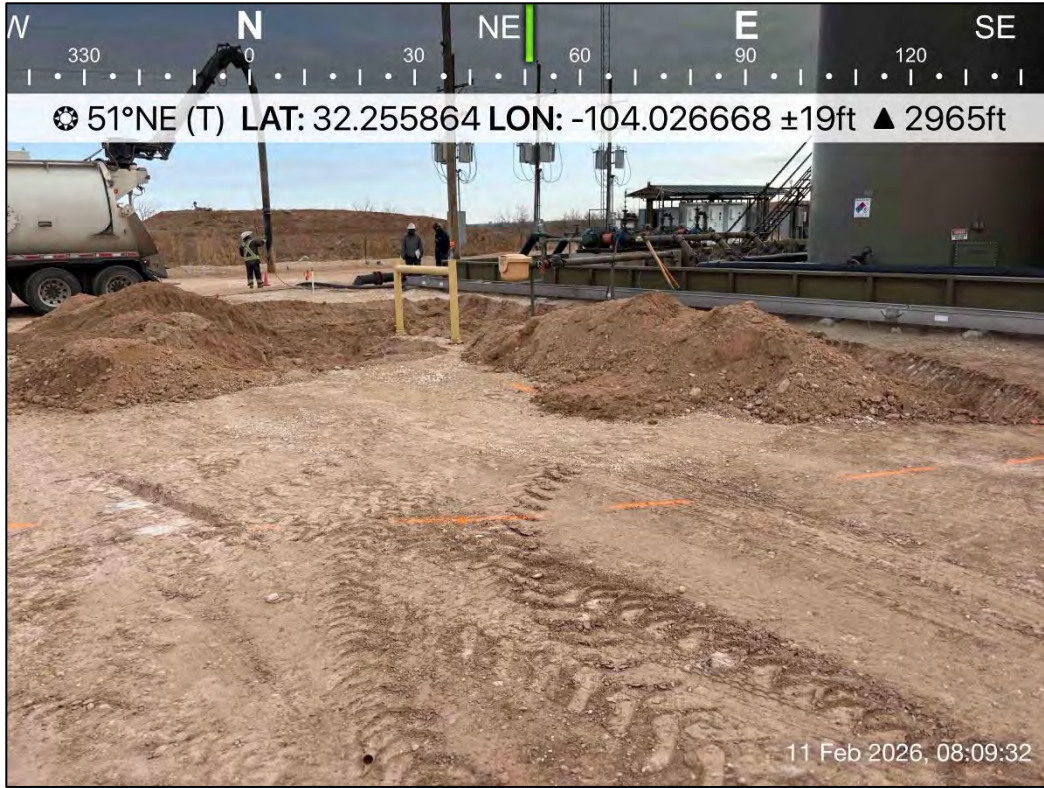
PHOTO 9: Northeastern view during excavation activities. 2/11/2026
