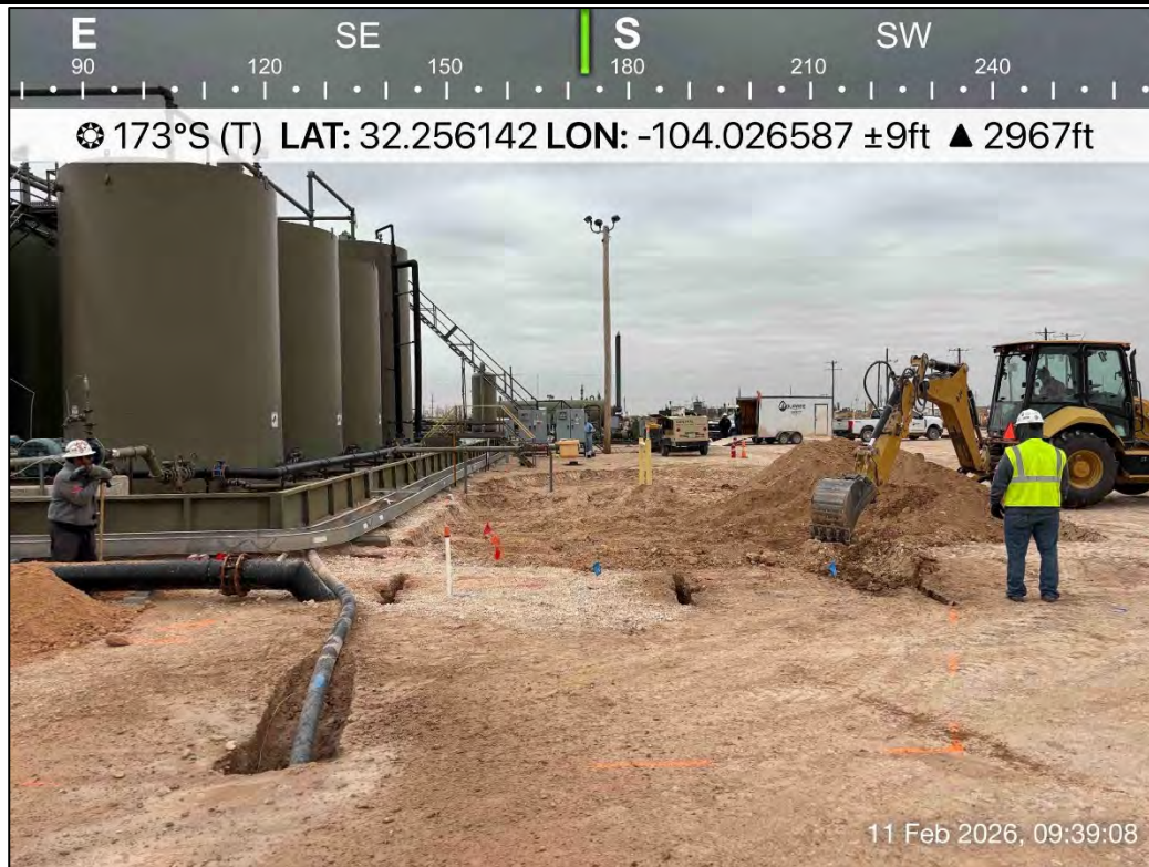
PHOTO 10: Southern view during excavation activities. 2/11/2026
