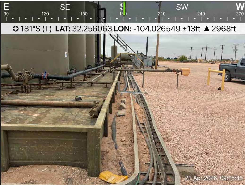
PHOTO 18: Southern view outside of containment during liner inspection activities. 4/21/2026
