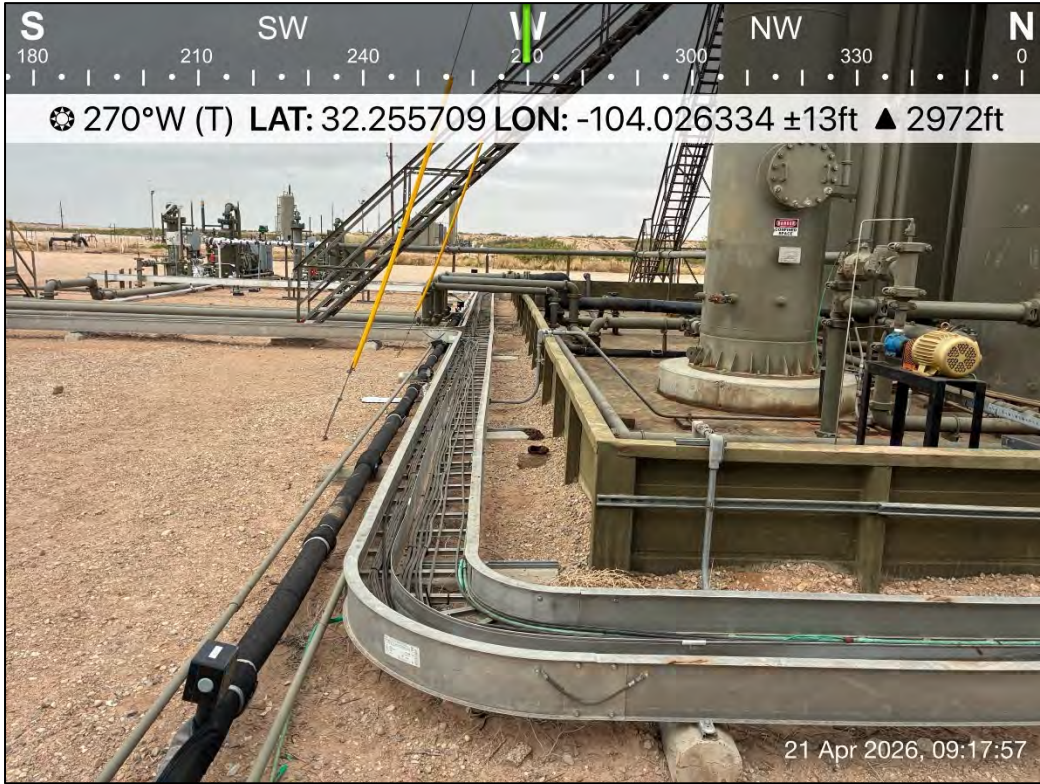
PHOTO 21: Western view outside of containment during liner inspection activities. 4/21/2026
