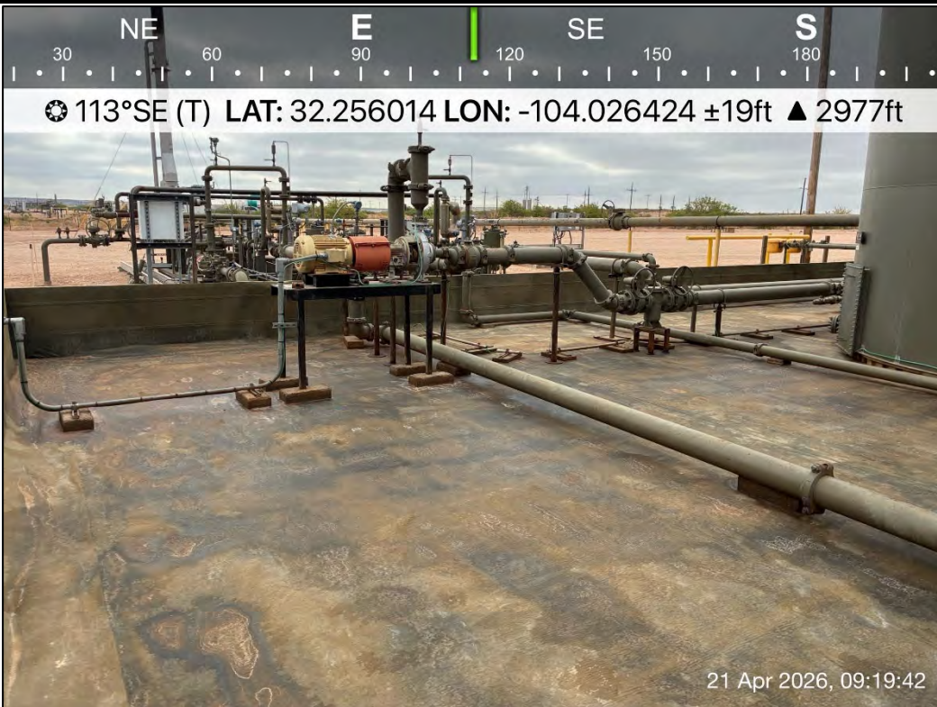
PHOTO 32: Southeastern view during liner inspection activities. 4/21/2026
