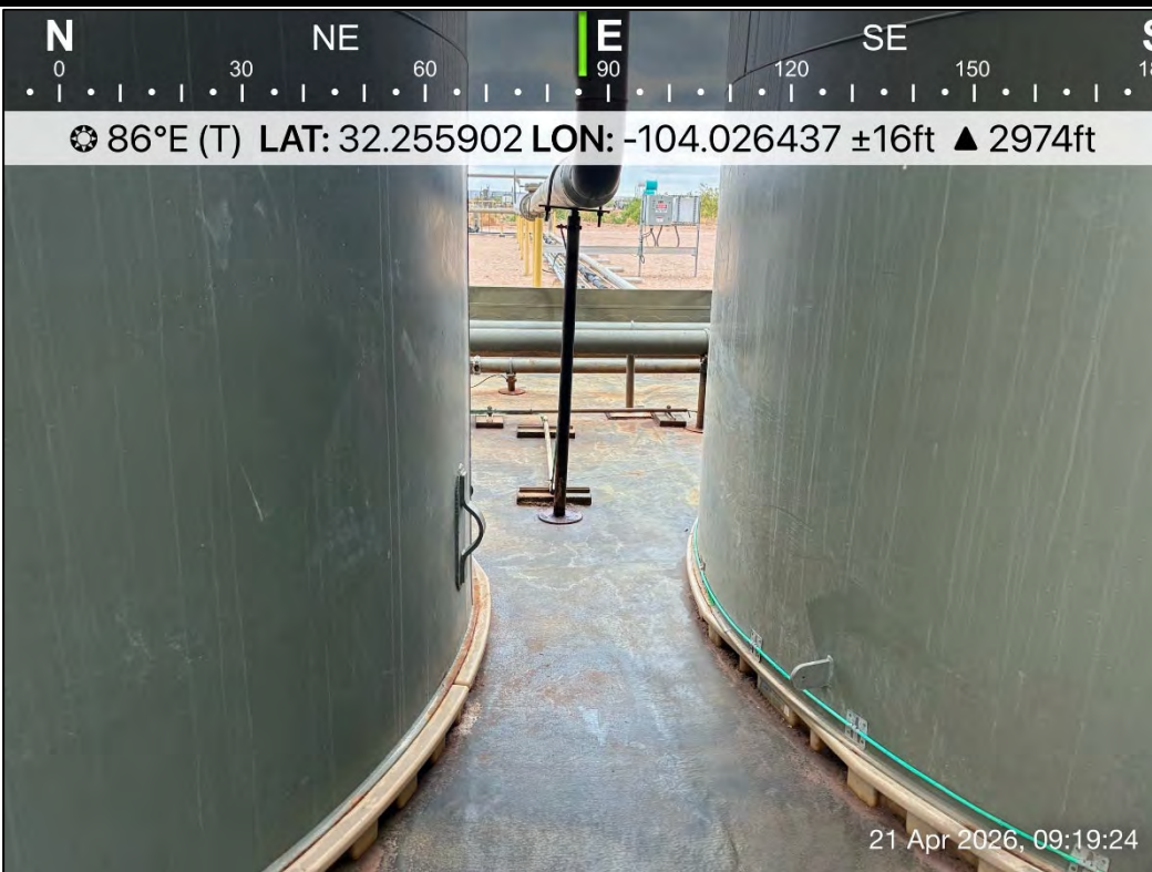
PHOTO 30: Eastern view during liner inspection activities. 4/21/2026
