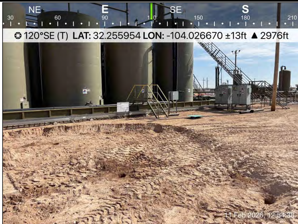
PHOTO 12: Southeastern view of excavation extent. 2/11/2026
