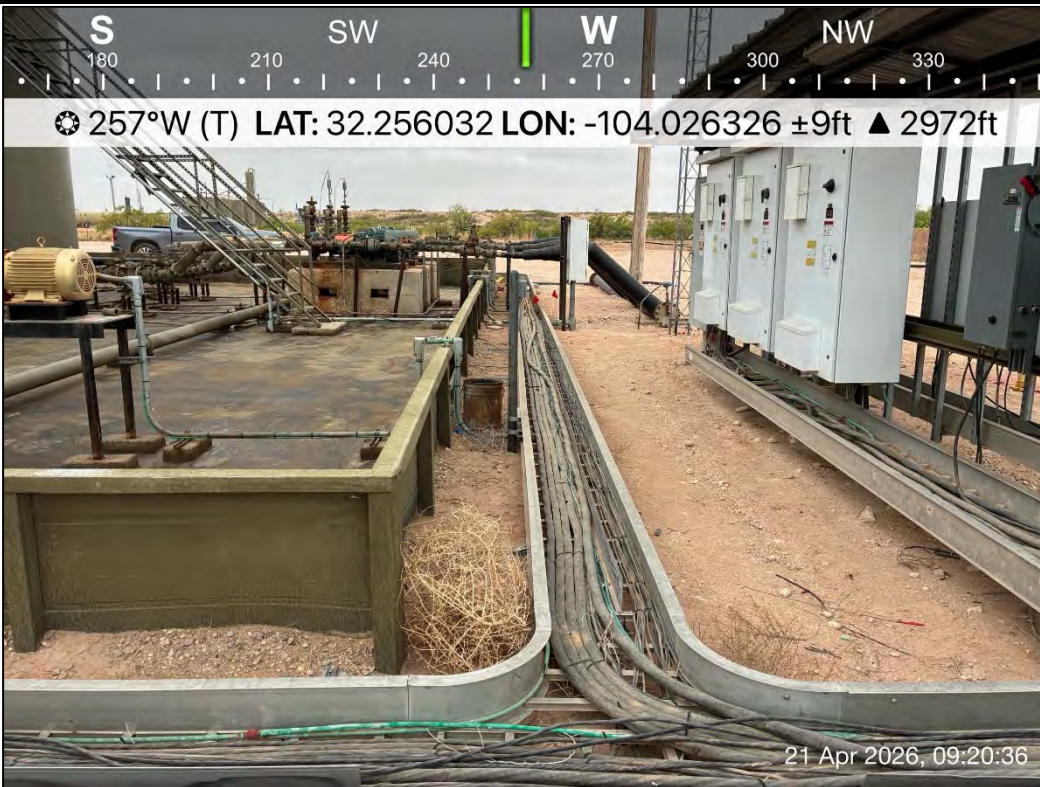
PHOTO 22: Southwestern view outside of containment during liner inspection activities. 4/21/2026
