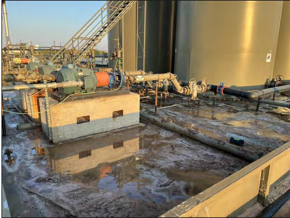
PHOTO 1: Southeastern view during initial site assessment. 8/25/2025
