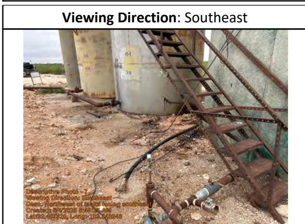
Northwest of tanks facing southeast.
