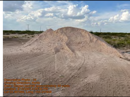
Staged backfill approximately 40 yards
