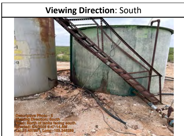
North of tanks facing south.
