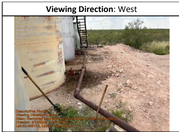
Removed asphaltic material from inside tank battery
