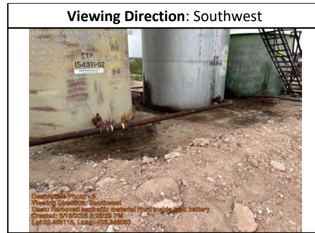
Removed asphaltic material from inside tank battery
