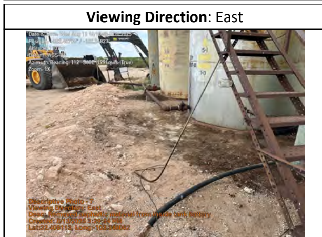
Removed asphaltic material from inside tank battery
