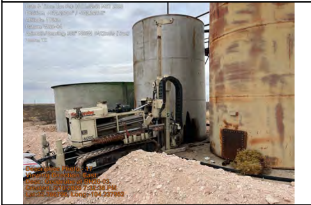
Geoprobe at BH26-03.
