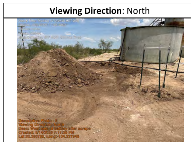
West side of battery after scrape
