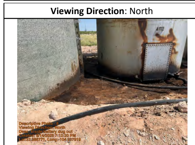
Inside battery dug out
