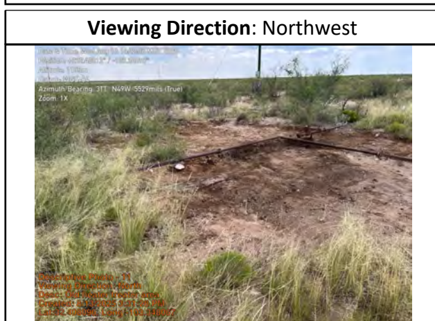
Old heater treater area
