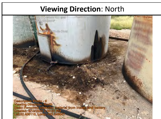
Removed asphaltic material from inside tank battery
