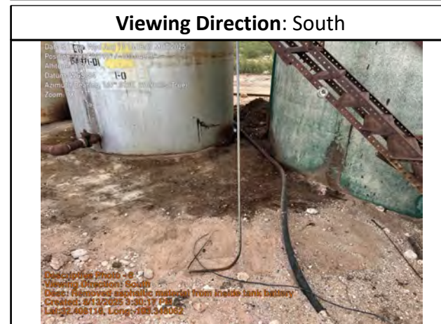
Removed asphaltic material from inside tank battery
