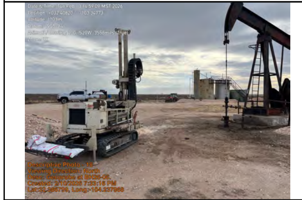
Geoprobe at BH26-06.
