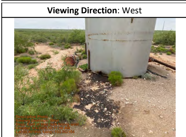
East of east tank facing west.
