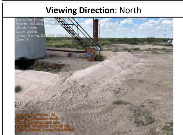
Repaired east berm
