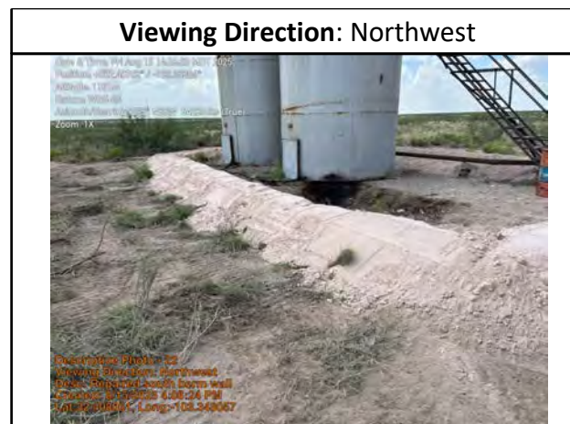
Repaired south berm
