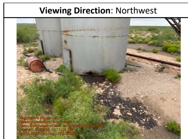
Southeast of east tank facing northwest.
