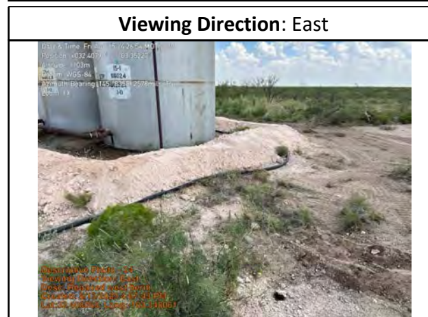
Repaired west berm
