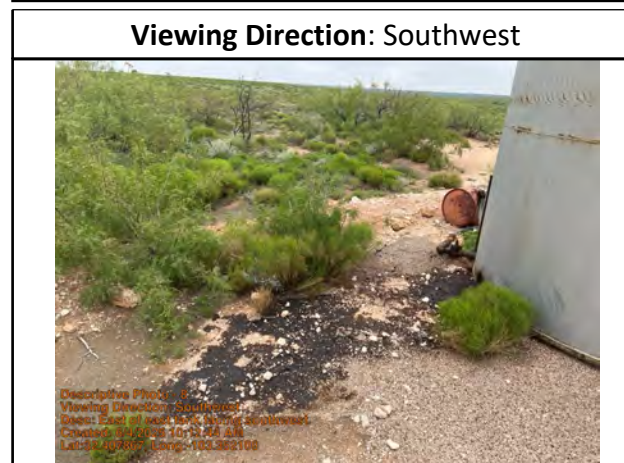
East of east tank facing southwest.
