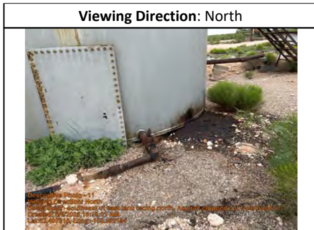
South-southeast of east tank facing north. Asphalt cropped out from base beneath tanks.
