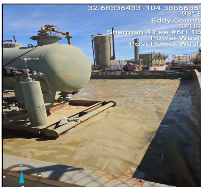
Photo taken post powerwash facing east.
