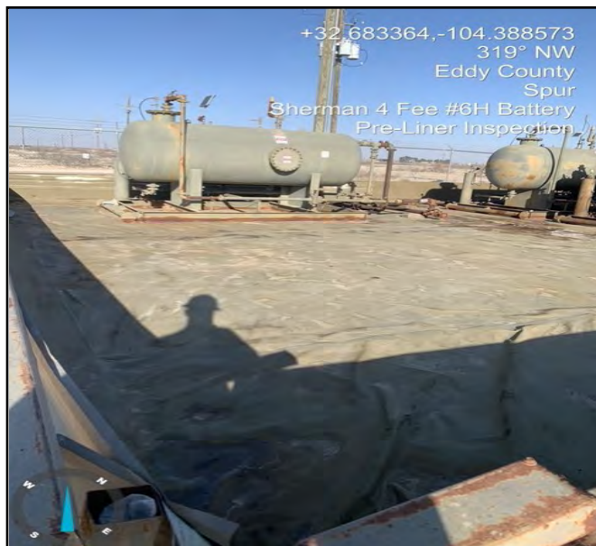
Photograph taken during initial assessment facing northwest.
