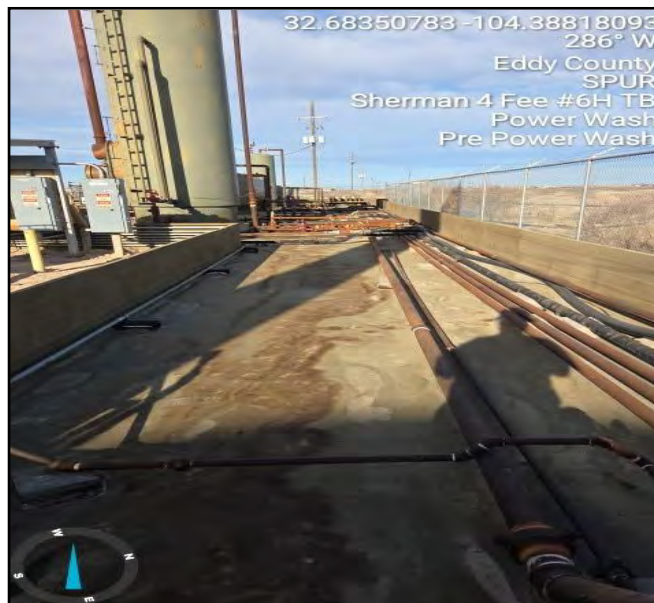
Photograph taken pre powerwash facing west.
