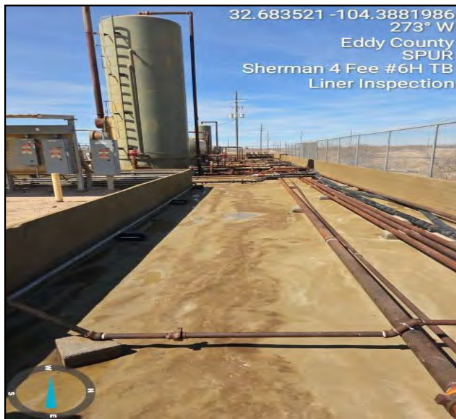
Photograph taken during the Liner Inspection facing west.
