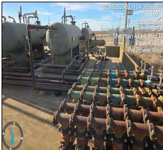
Photograph taken pre powerwash facing south.
