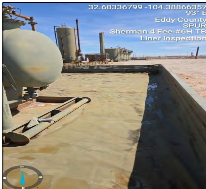
Photograph taken during the Liner Inspection facing east.
