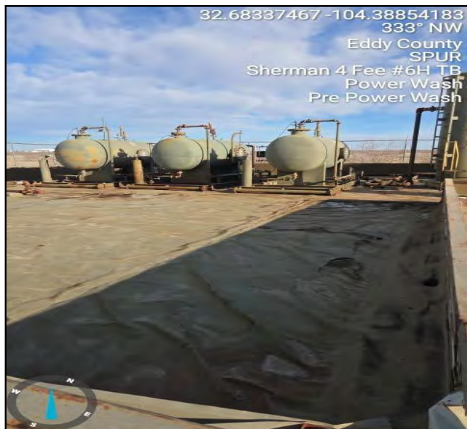
Photograph taken pre powerwash facing northwest.
