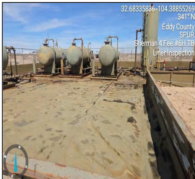
Photograph taken during the Liner Inspection facing north.
