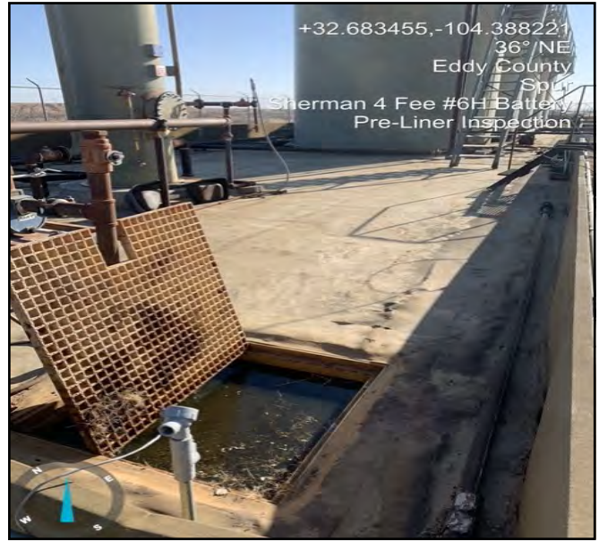
Photograph taken during initial assessment facing northeast.
