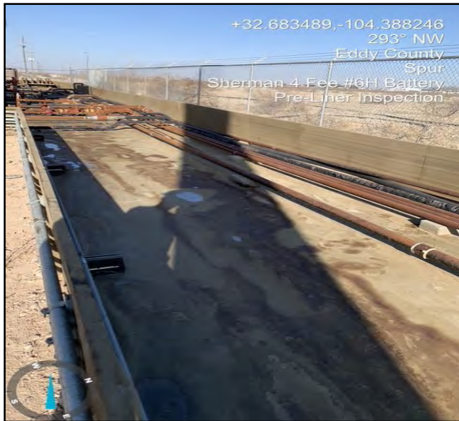
Photograph taken during initial assessment facing northwest.
