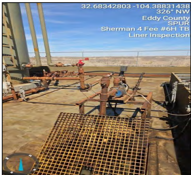
Photograph taken during the Liner Inspection facing northwest.
