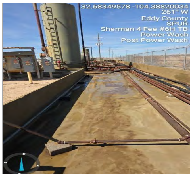
Photo taken post powerwash facing west.
