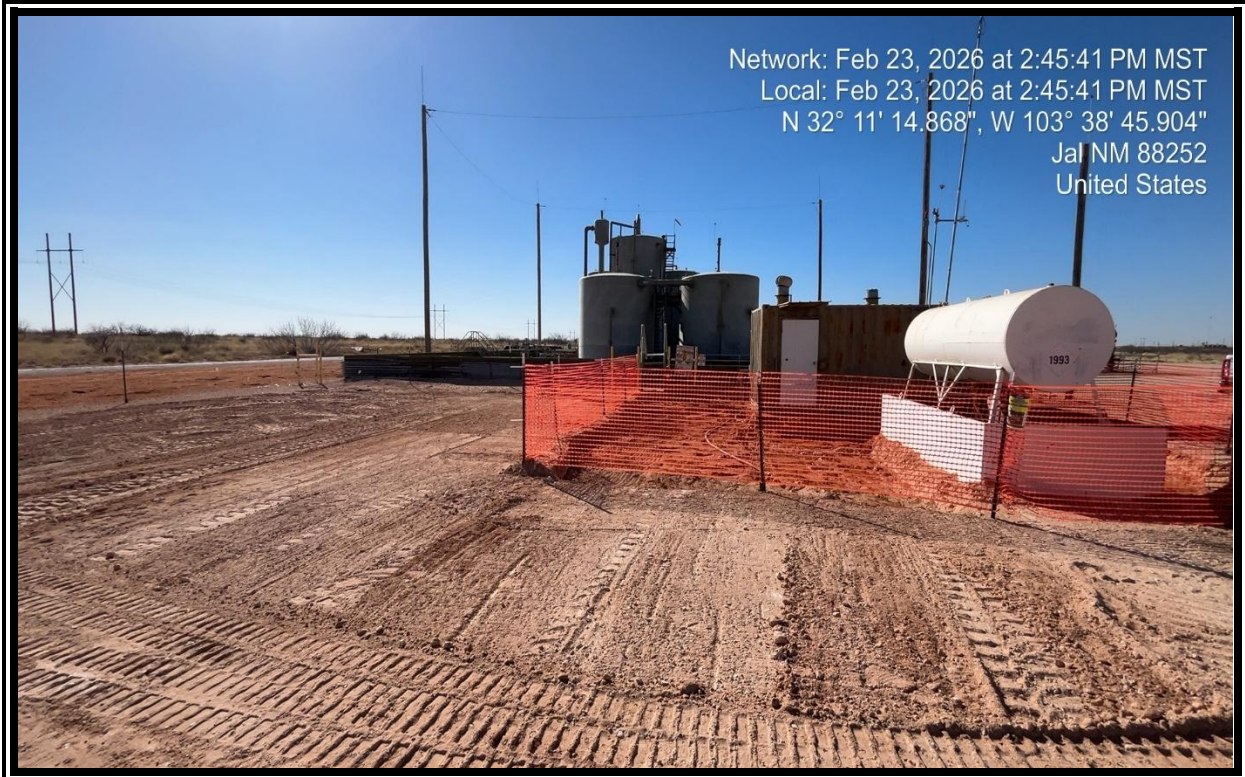
View of the site during excavation activities.
