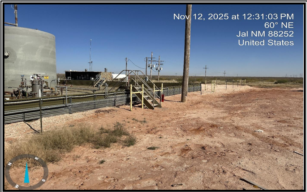
View of the site during assessment activities.
