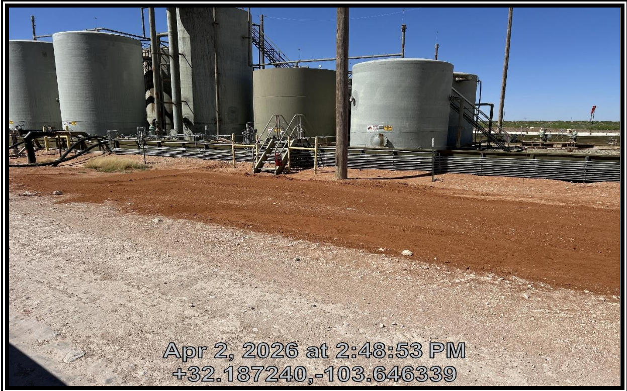
View of the site following remediation activities.
