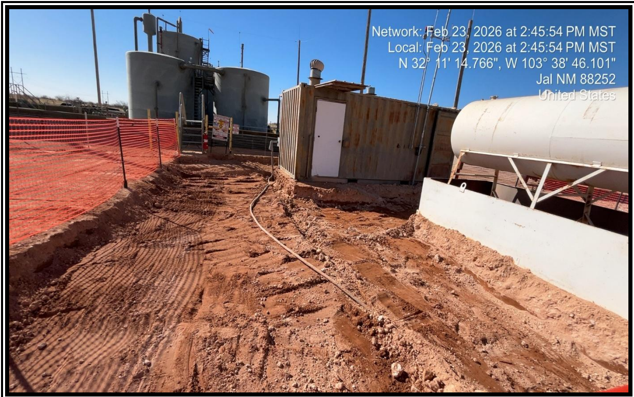
View of the site during excavation activities.
