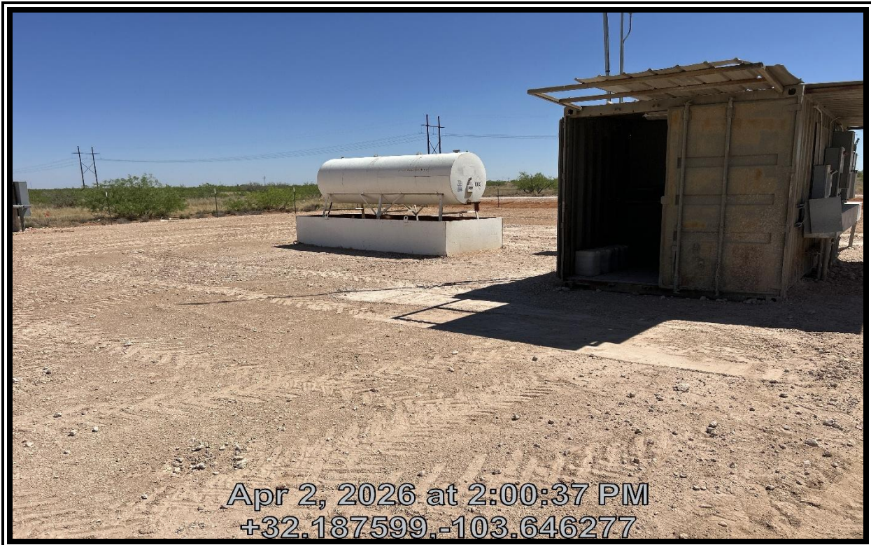
View of the site following remediation activities.
