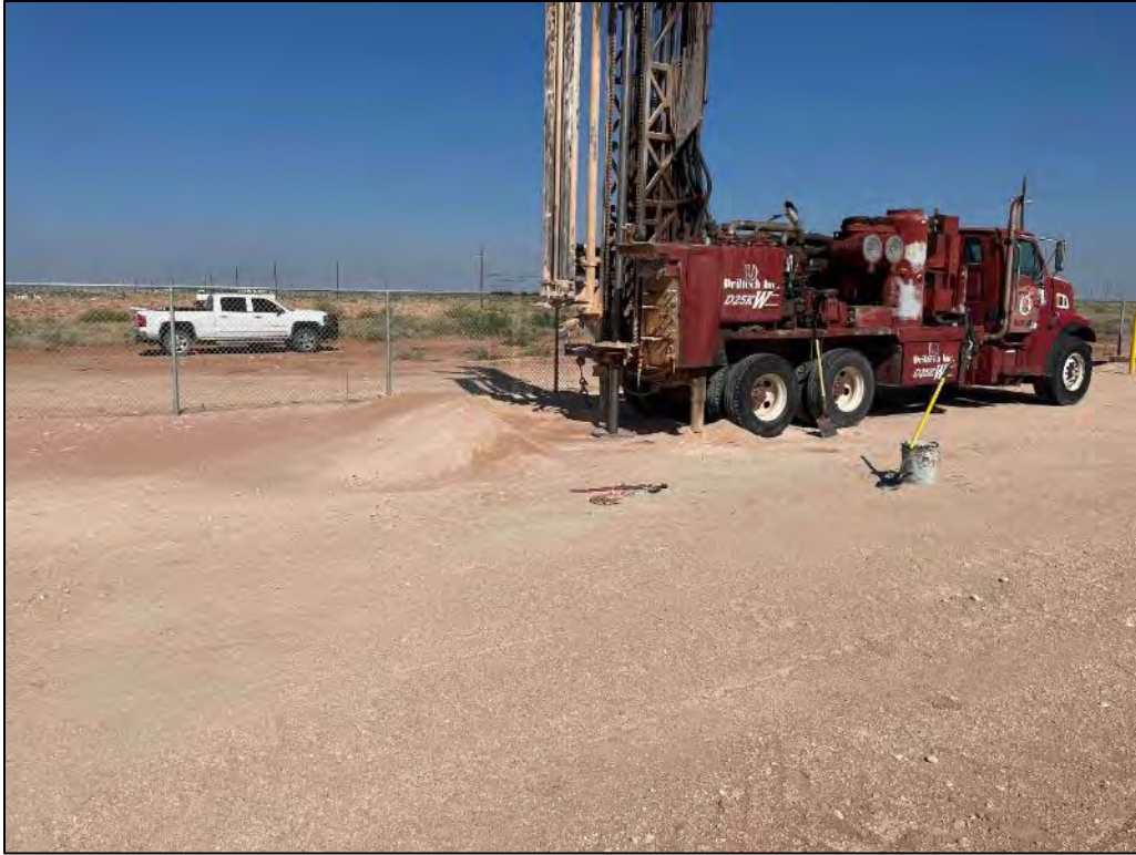
PHOTO 7: View of the borehole being drilled facing northwest. 8/29/23
