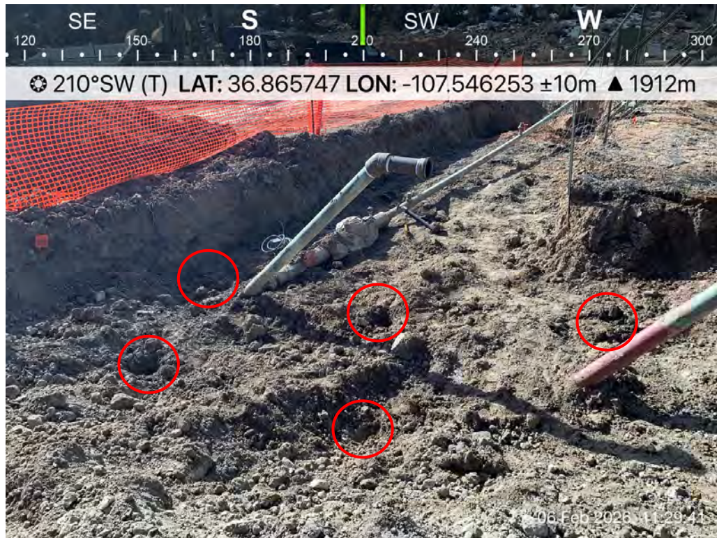
Photo 18: SS17 collected as a 5pct sample from the base of the POR excavation.
