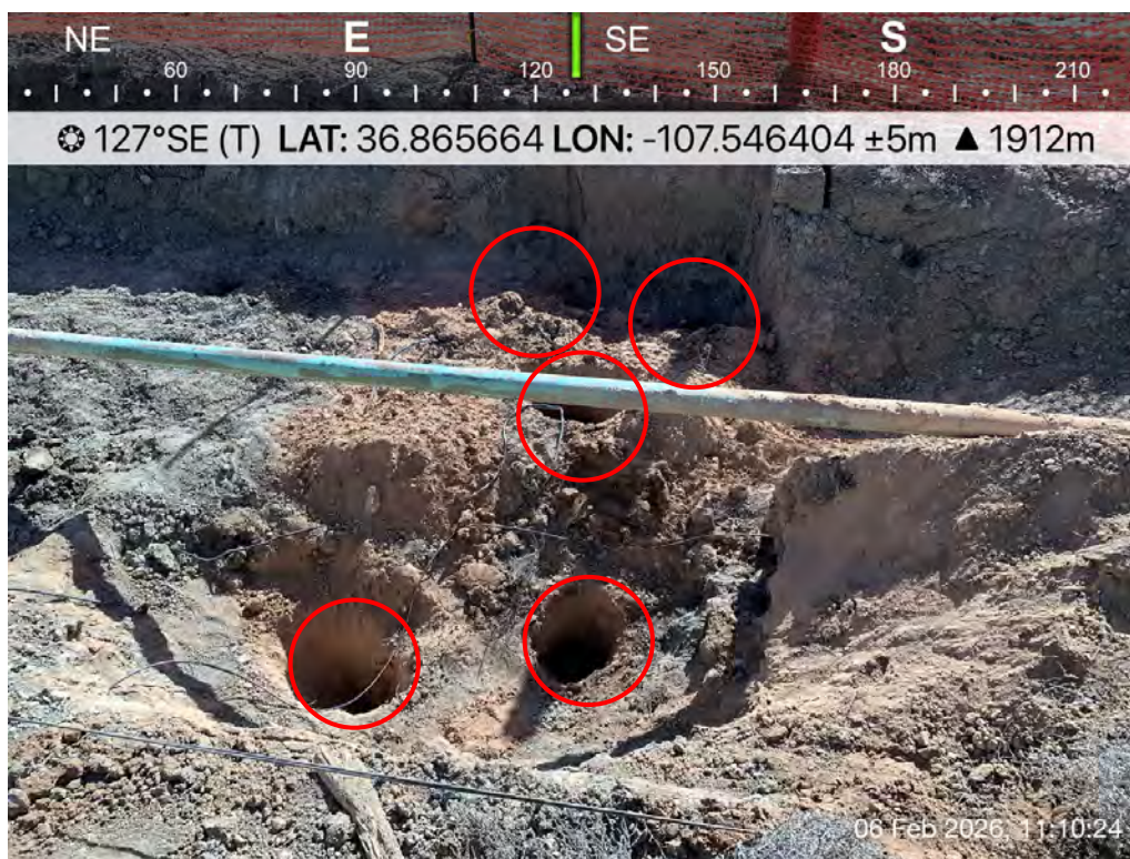
Photo 13: SS12 collected as a 5-point composite (5pct) sample from the base of the POR excavation.
