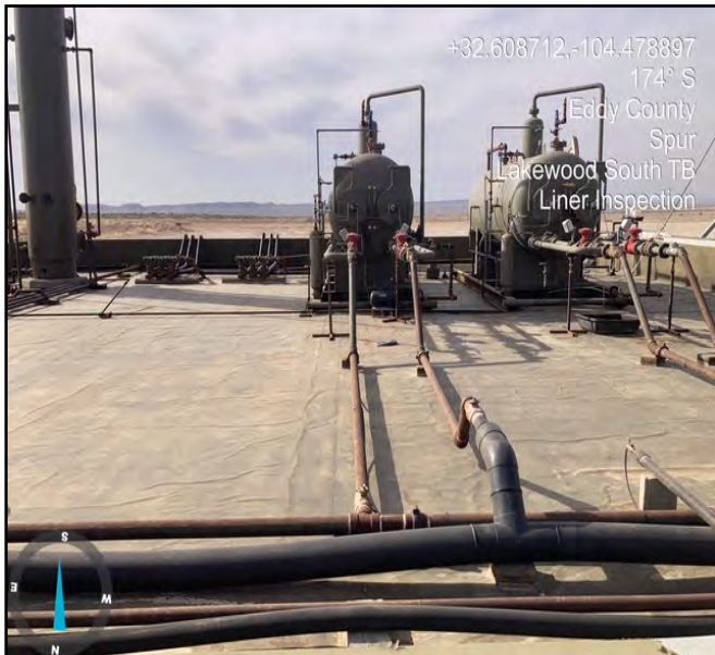
Photograph taken during initial assessment facing south.
