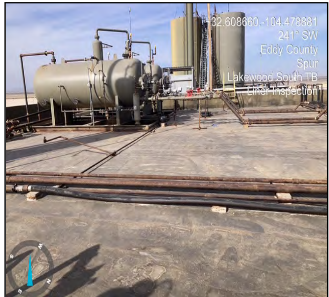
Photograph taken during initial assessment facing southwest.
