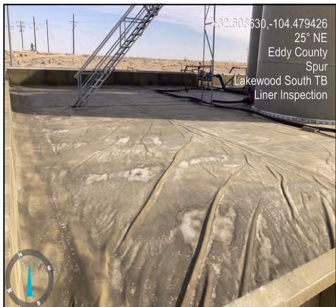
Photograph taken during initial assessment facing northeast.
