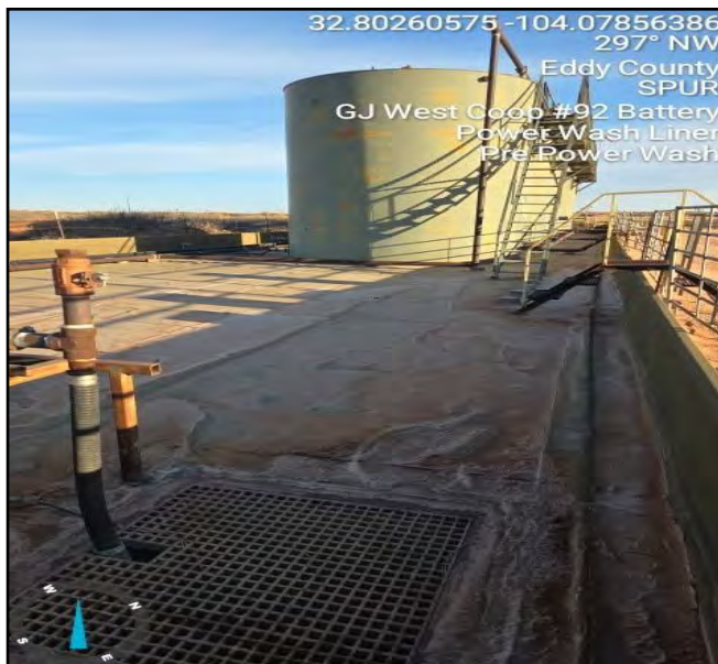
Photograph taken pre powerwash facing northwest.
