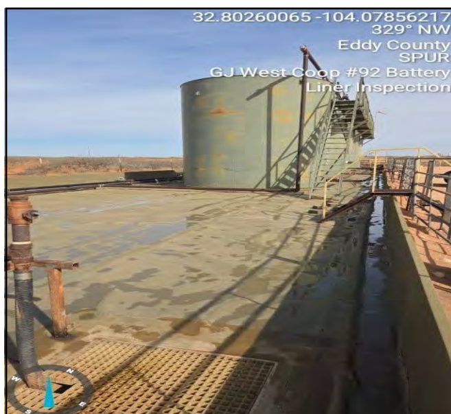
Photograph taken during Liner Inspection facing northwest.
