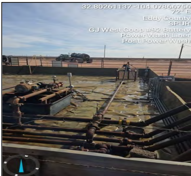
Photograph taken post powerwash facing east.
