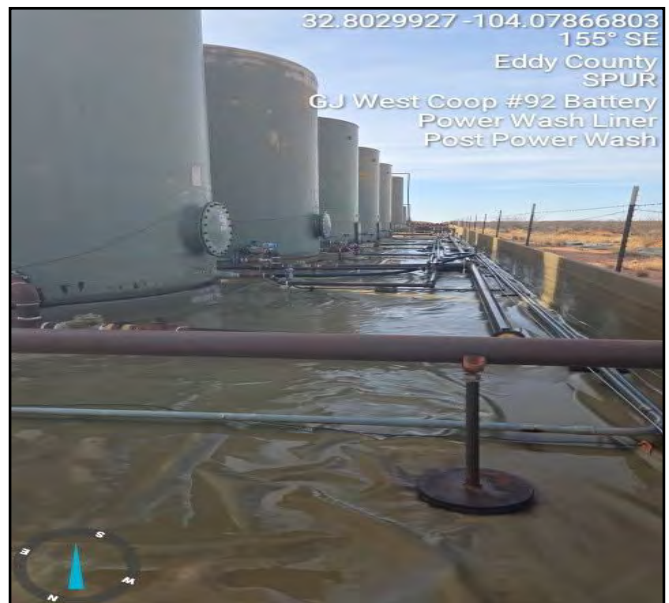
Photograph taken post powerwash facing southeast.
