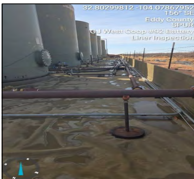
Photograph taken during Liner Inspection facing southeast.
