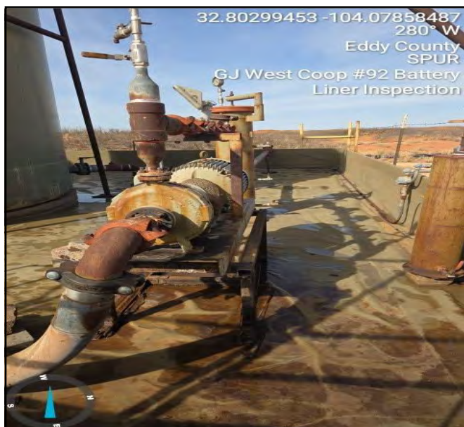
Photograph taken during Liner Inspection facing west.
