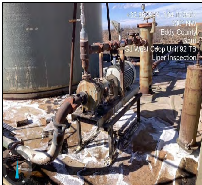
Photograph taken during initial spill release facing northwest.
