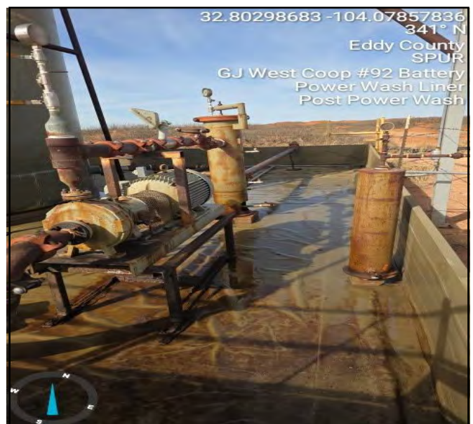
Photograph taken post powerwash facing north.
