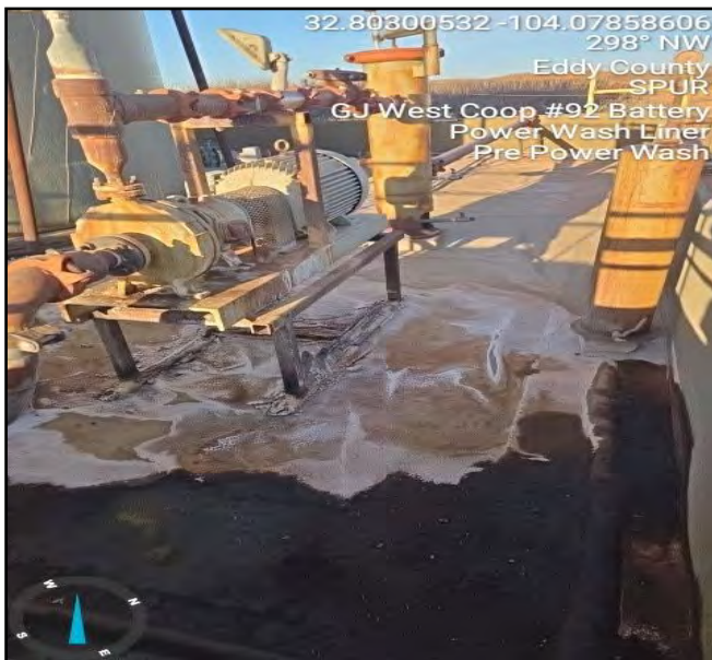
Photograph taken pre powerwash facing northwest.
