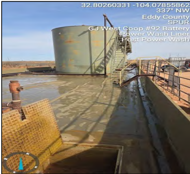
Photograph taken post powerwash facing northwest.
