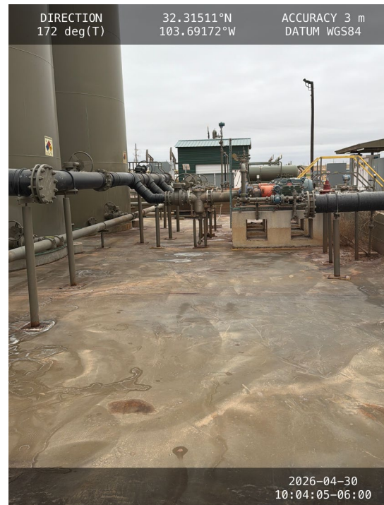
Photo 4 View of containment towards south.
