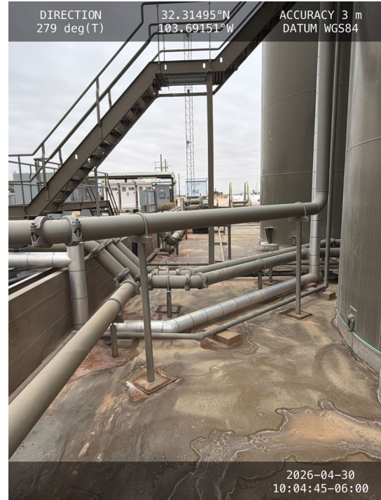
Photo 10 View of containment towards west.
