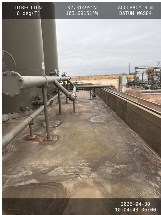
Photo 11 View of containment towards north.
