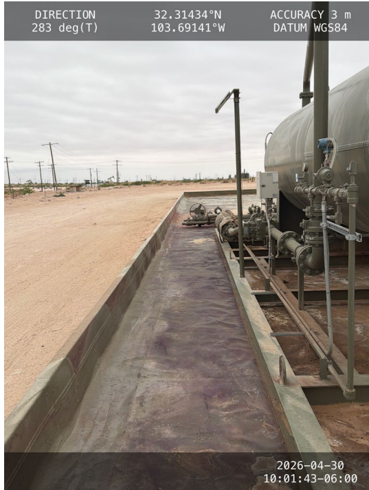
Photo 9 View of northwest corner of containment.
