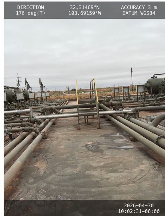
Photo 16 View of the central area towards south.
