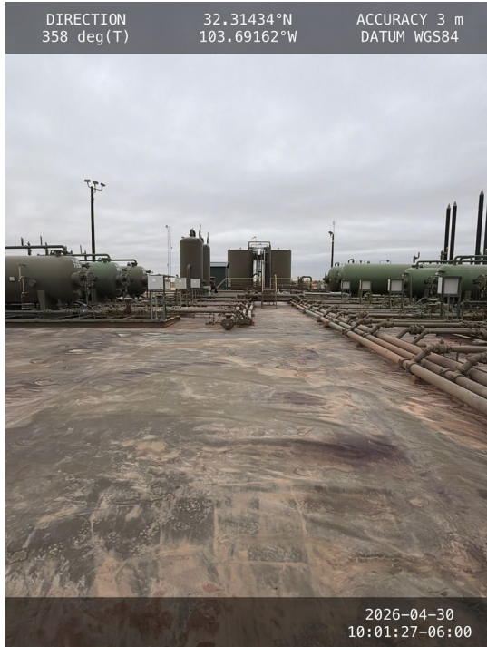
Photo 13 View of central containment towards north.
