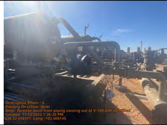
Release point from piping coming out of V-109 84H identified
