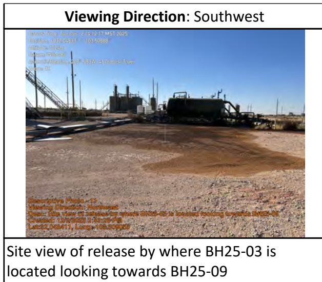
Site view of BH25-09. Attempted to collect a 4ft and 5ft sample however was hitting refusal with auger at 3.5ft
