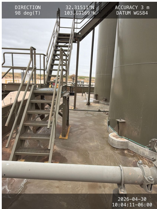
Photo 3 View of containment towards east.
