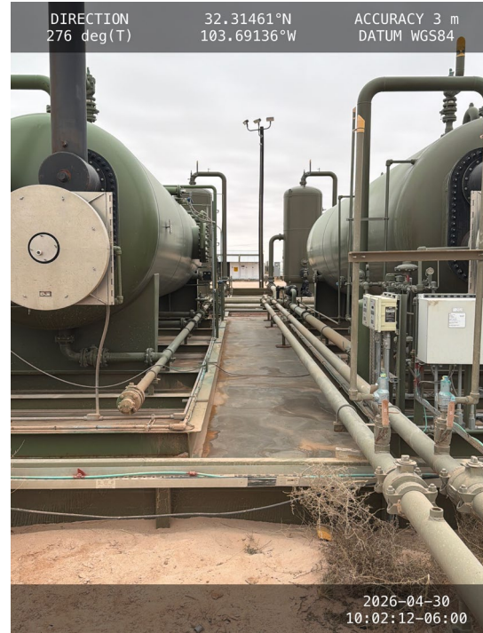
Photo 13 View of the secondary containment towards west.
