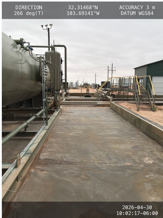
Photo 15 View of containment towards west.
