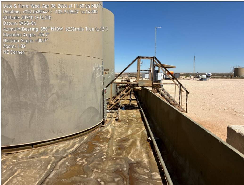
PHOTO 19: Northwestern view during liner inspection activities. 4/8/2026
