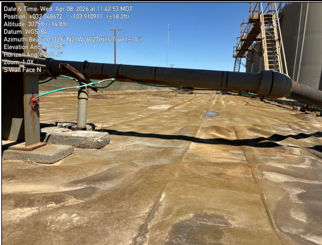
PHOTO 10: Northwestern view during liner inspection activities. 4/8/2026
