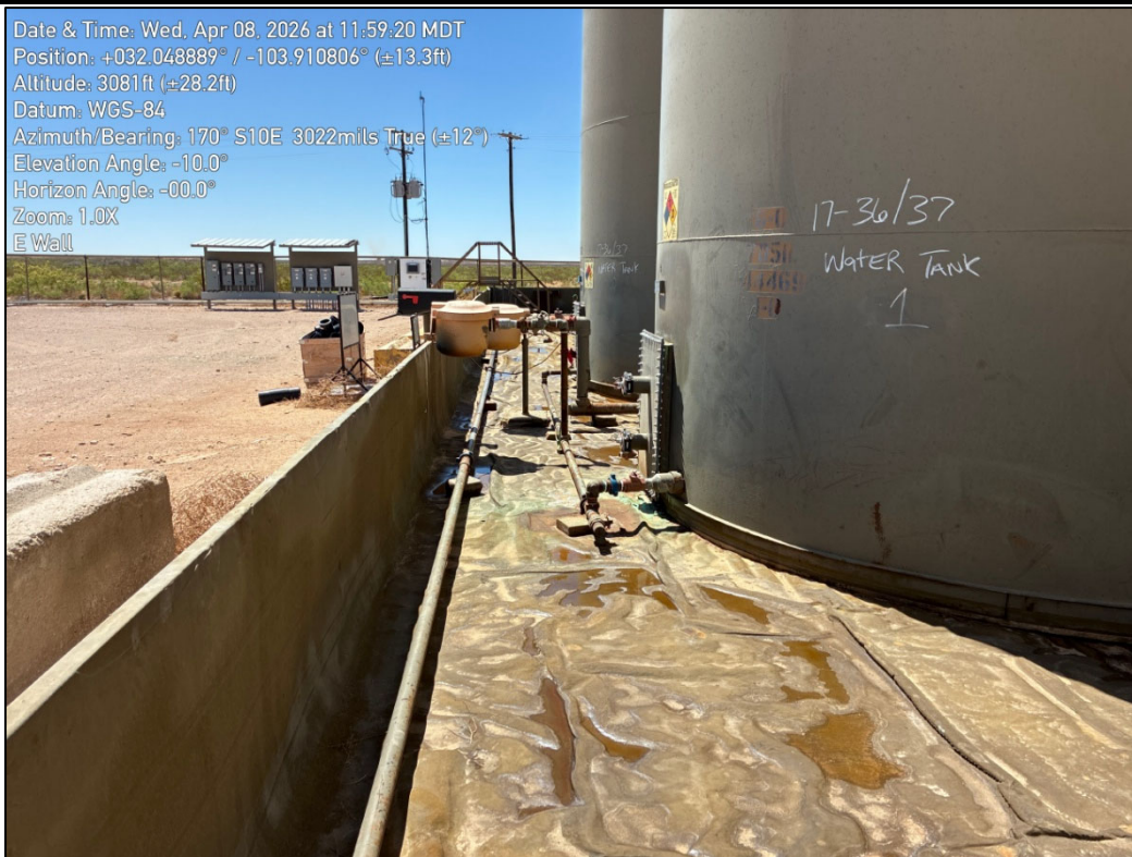
PHOTO 16: Southeastern view during liner inspection activities. 4/8/2026
