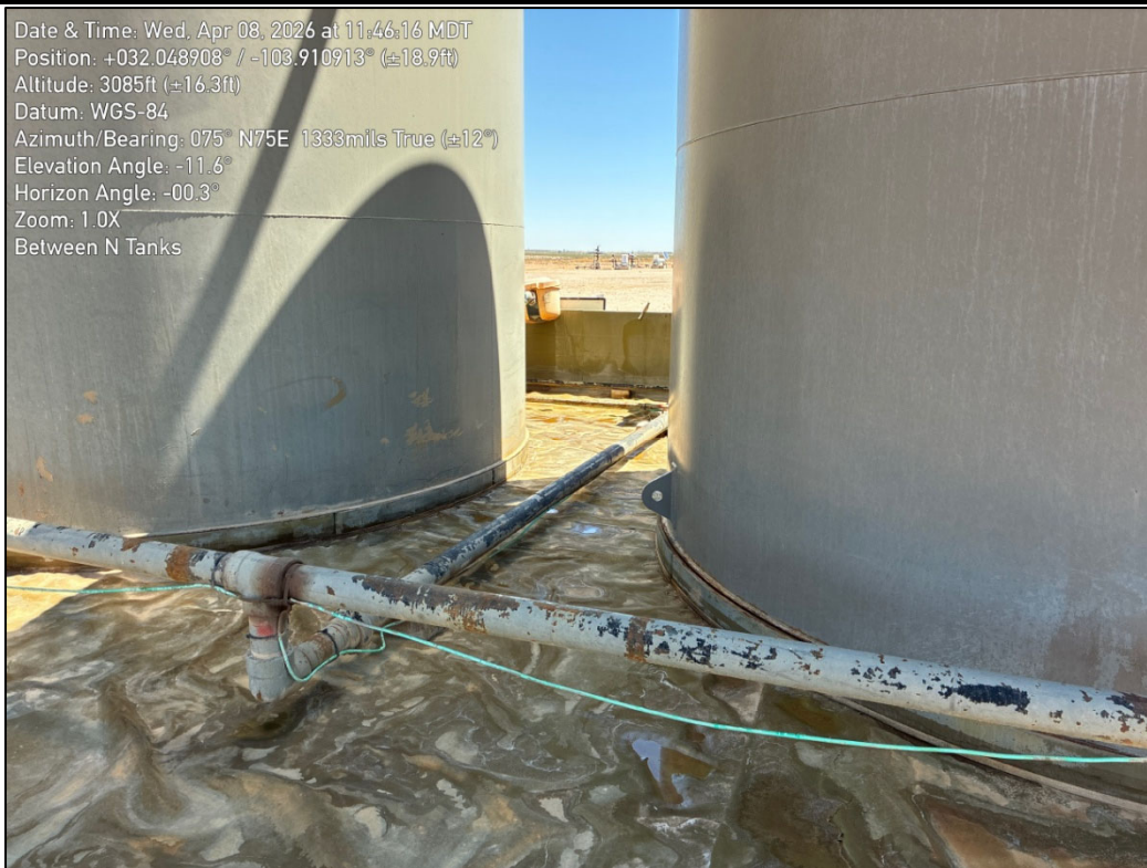
PHOTO 12: Northeastern view during liner inspection activities. 4/8/2026
