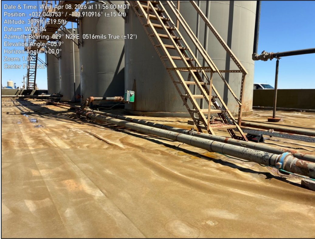
PHOTO 17: Northeastern view during liner inspection activities. 4/8/2026
