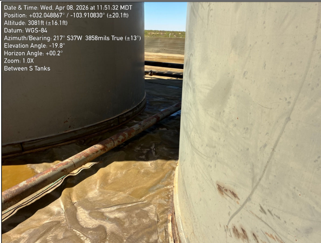
PHOTO 14: Southwestern view during liner inspection activities. 4/8/2026
