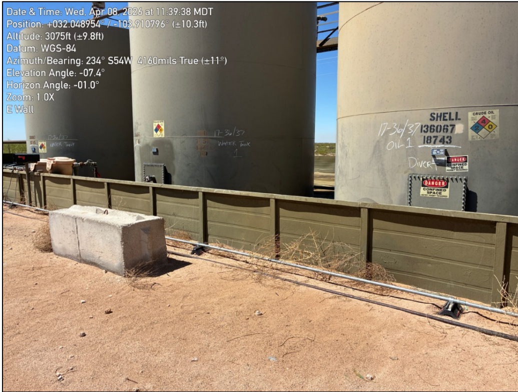
PHOTO 9: Southwestern view outside of containment during liner inspection activities. 4/8/2026
