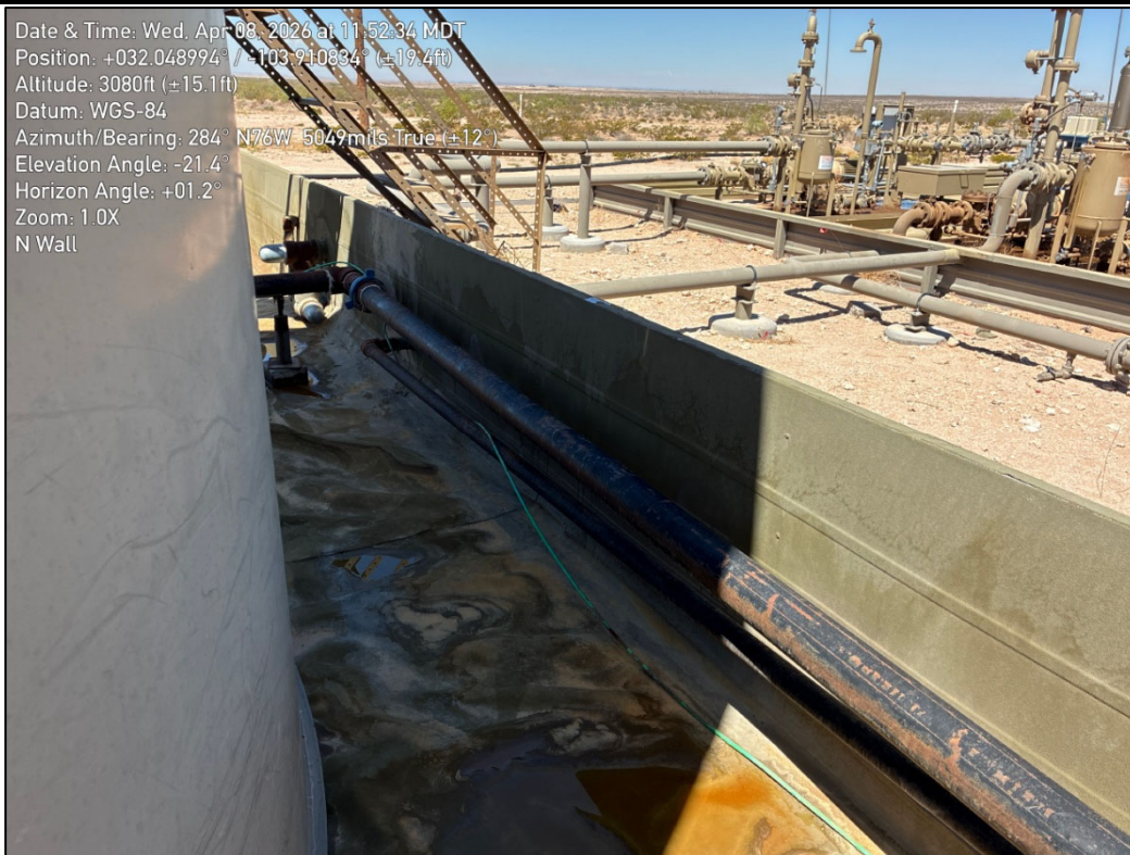
PHOTO 18: Northwestern view during liner inspection activities. 4/8/2026
