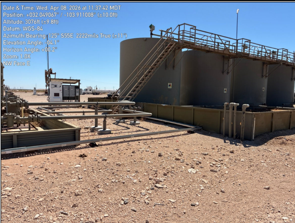
PHOTO 8: Southeastern view outside of containment during liner inspection activities. 4/8/2026
