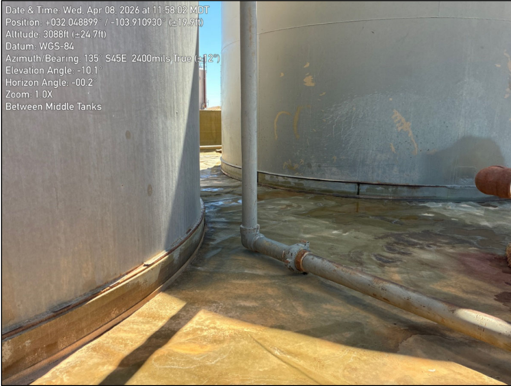
PHOTO 15: Southeastern view during liner inspection activities. 4/8/2026
