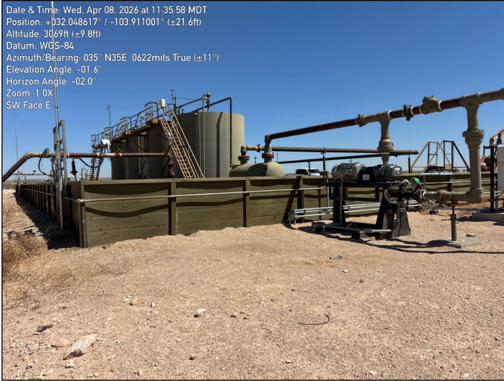
PHOTO 5: Northeastern view outside of containment during liner inspection activities. 4/8/2026
