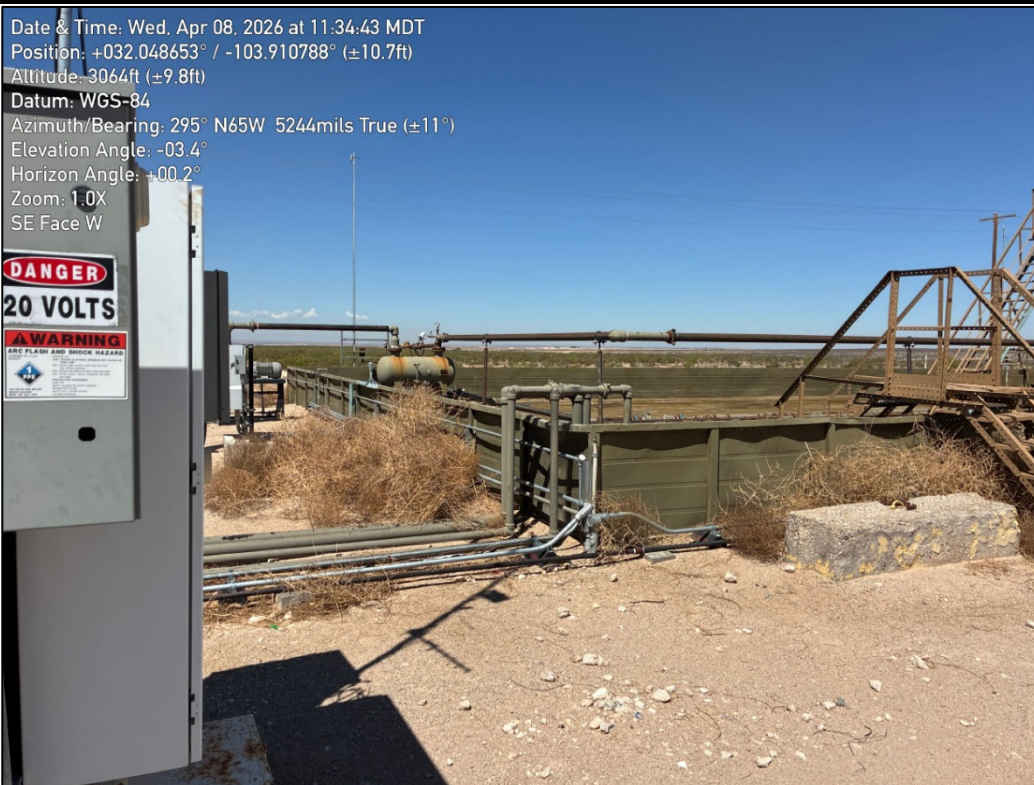
PHOTO 4: Northwestern view outside of containment during liner inspection activities. 4/8/2026
