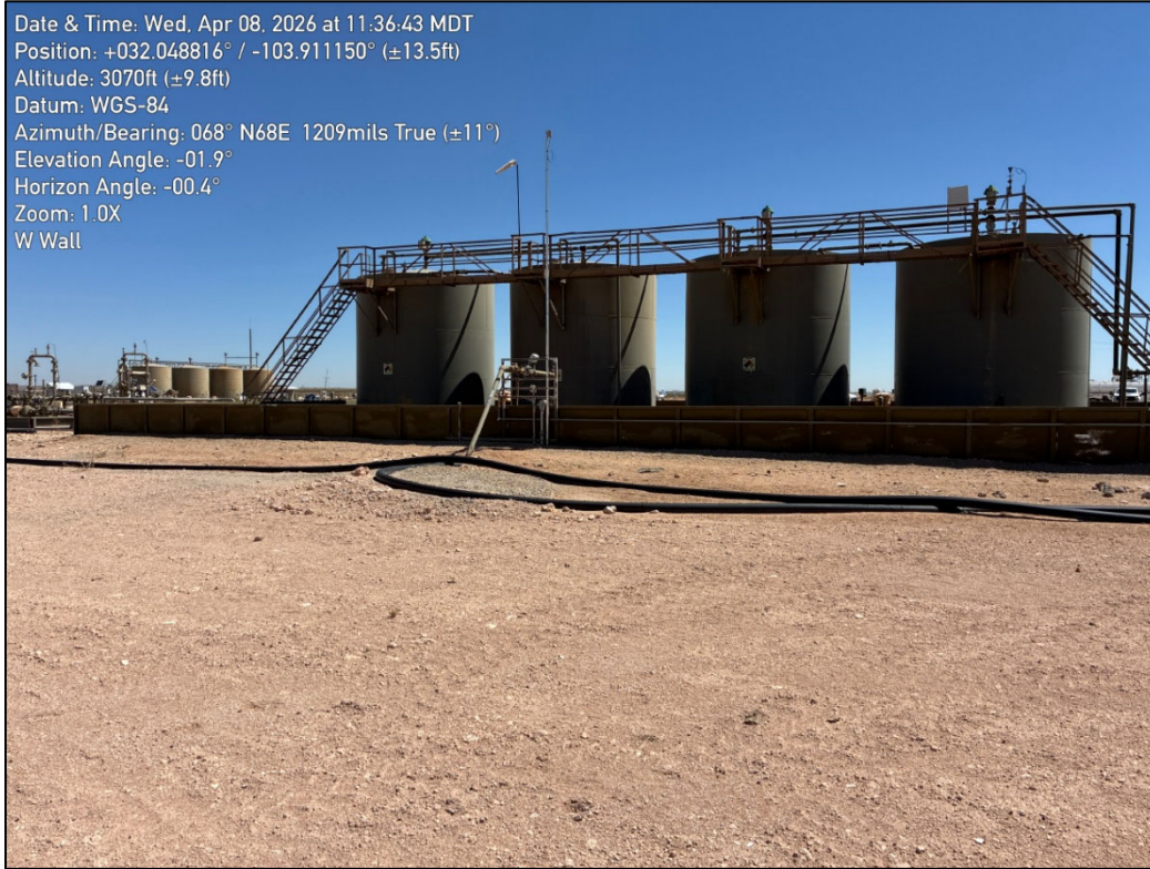
PHOTO 7: Northeastern view outside of containment during liner inspection activities. 4/8/2026
